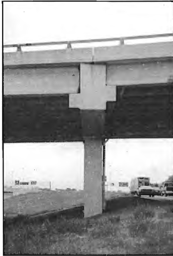
Figure 5.12 A change in superstructure depth highlighted by the awkwardly shaped bent cap end
