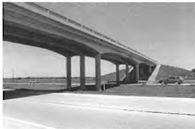
Figure 4.4 Individual columns supporting individual cast-in-place continuous beams
