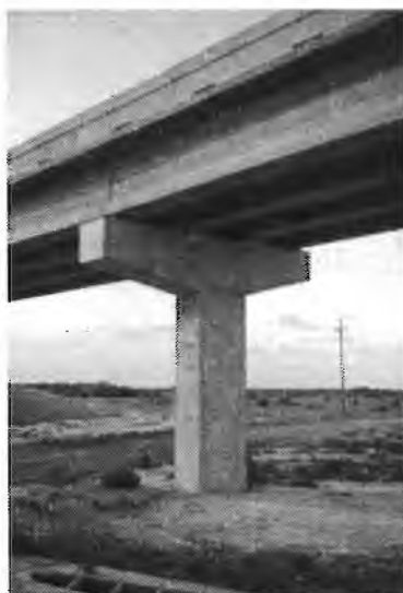
A rectangular column and prismatic cap (a) and a rounded column joining a prismatic cap (b).
