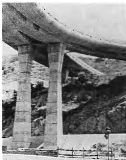
(a) These tall piers are more fixed at the base than at transverse the top. Under critical lateral loads, the point of inflection is located at about two-thirds the height from the base, allowing the columns to taper in at that location of minimum moment. [58]
