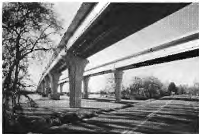
Figure 4.48 Vertical relief enhances the slenderness of this pier.
