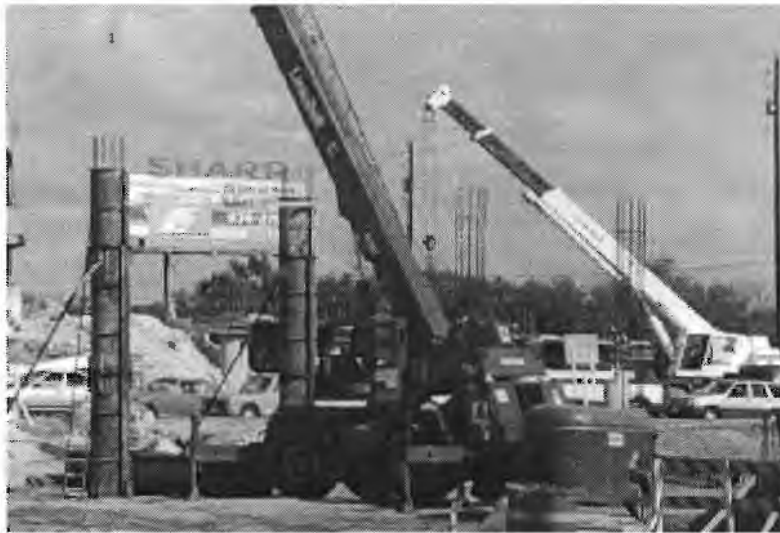
Figure 1.3 Extensive on-site equipment for cast-in-place multicolumn bents
