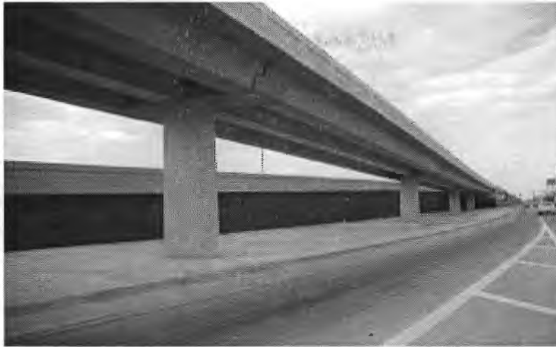
Figure 4.15 A hammerhead bent cap fully integrated into the depth of the superstructure through the use of dapped girders
