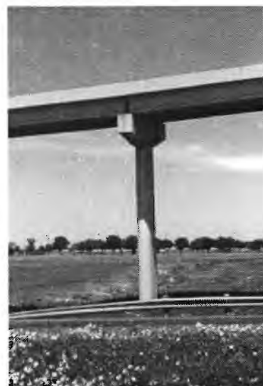
A rectangular column and prismatic cap (a) and a rounded column joining a prismatic cap (b).
