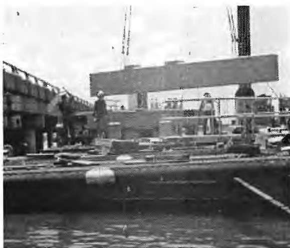
Figure 2.5 Precast pile caps for the Redfish Bay low water crossing. A minimal amount of cast-in-place concrete is used in making cap to pile connections.
