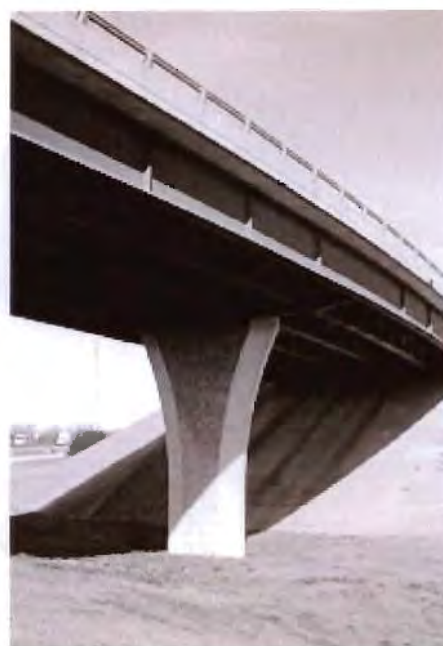
Figure 4.55 An elegantly tapered pier exposed aggregate used to accent slenderness; however, a disconcerting overall design—see Figure 4.23
