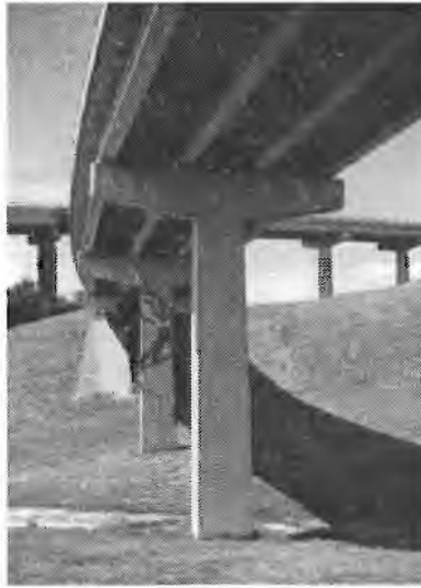
The tapered cap and column of this hammerhead bent is structurally expressive of the increased moment resistance required at the cap/column intersection and at the column base under critical loads
