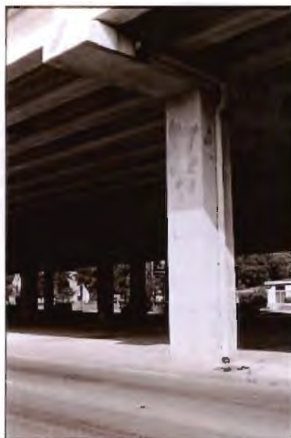
Figure 4.58 Unattractive peeling of painted concrete
