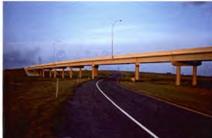
Figure 4.57 Concrete painted with an earthtone to integrate with the landscape
