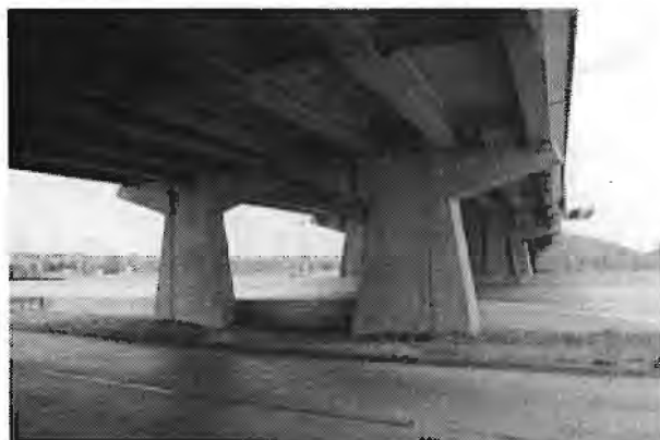
Extreme tapering in short substructure units exaggerates the flow of forces and appears contrived.
