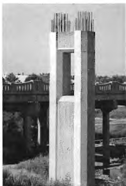
Figure 5.19 A windowed pier under construction for US 67
