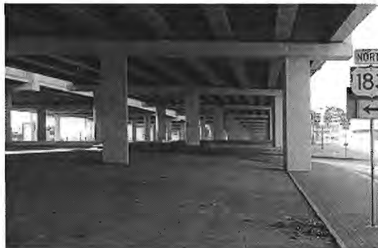
Figure 4.18 Rectangular columns joining a prismatic inverted-T cap
