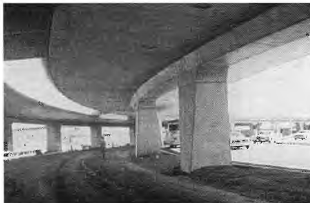
(b) The tapers in these piers vary in both the longitudinal and transverse directions. In the transverse direction, the columns are vertical cantilevers fixed at the base and pinned at the top. In the longitudinal direction, the columns are pinned at the base to relieve shrinkage and creep stresses in the post tensioned deck are "fixed" at the top to provide continuity between the super- and substructure. [58]
