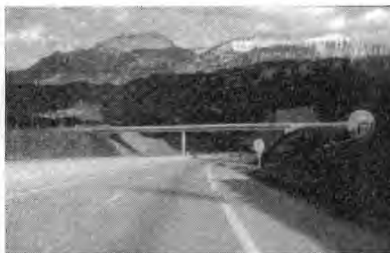
(b) A completed channel bridge
