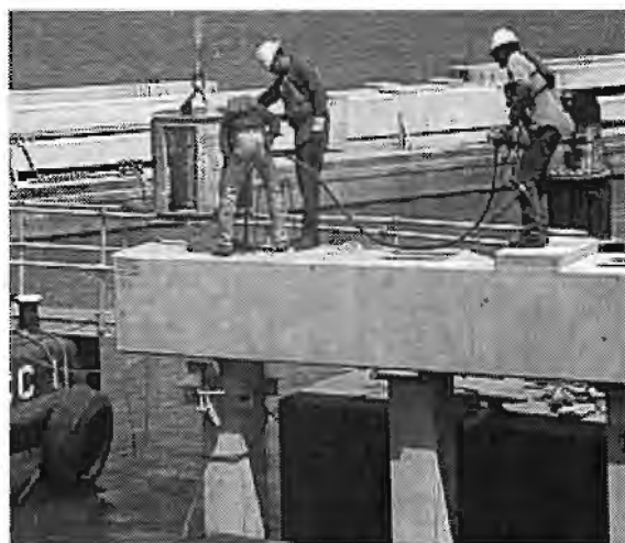
Figure 2.5 Precast pile caps for the Redfish Bay low water crossing. A minimal amount of cast-in-place concrete is used in making cap to pile connections.
