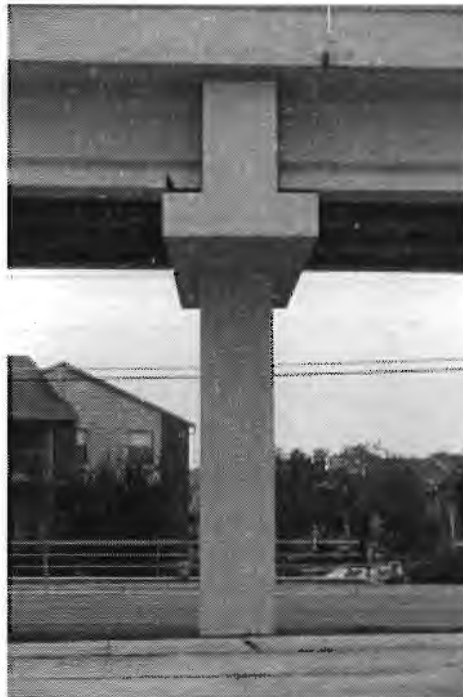
Figure 4.66 Balanced appearance of a column and bent cap stem of equal width
