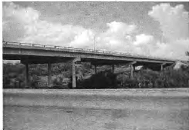
Figure 5.7 A precast prestressed concrete I-girder bridge crossing the Concho River
