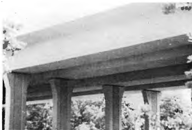
Figure 4.6 Individual columns supporting individual trapezoidal box girders
