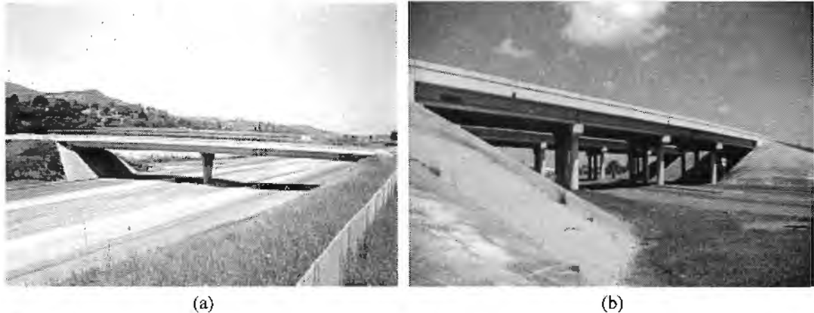
Figure 4.29 A simple tapered single support (a) is a more elegant solution than a series of multicolumn bents (b) for a standard overpass
