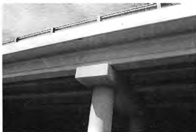
Figure 4.65 Inverted-T bent cap stem shaped to mimic the concrete I-girders it supports
