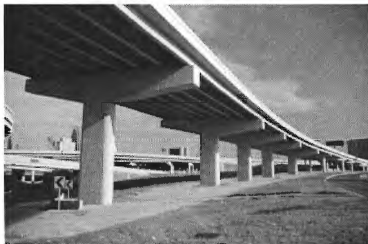
Figure 4.13 Hammerhead bents entirely underneath the superstructure
