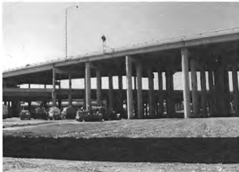
Figure 4.16 Cluttered multicolumn bents create "forests" of columns
