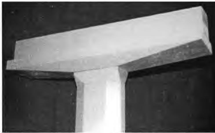
Figure 3.8 Column and cap visually integrated with flaring chamfers on the template segment of Proposal I
