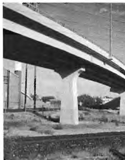
A flared column that stops short of the outer girders leaves the viewer with a sense of uneasiness about the support of the superstructure.
