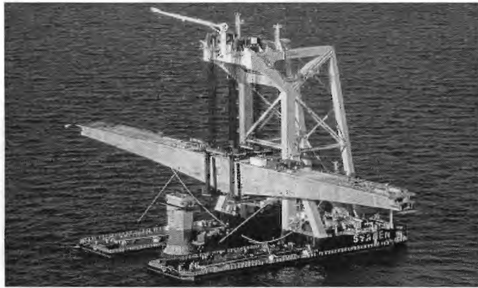
Figure 3.6 Placement of a 200 m (655 ft.) precast segmental girder for the Northumberland Strait crossing.[19] (Template segment is in position on top of the pier.)
