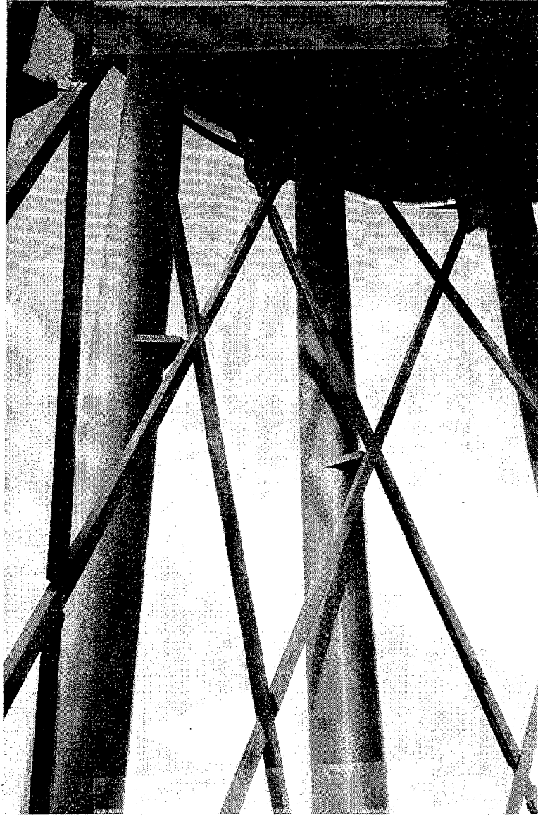
Photo 8: Seattle Public Utilities Magnolia Elevated Tank Seismic Upgrade
