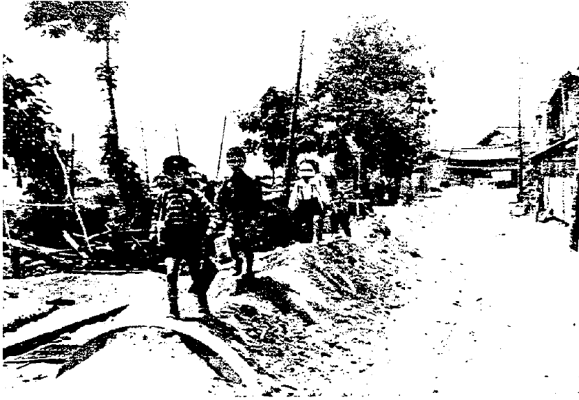
Photo 1 Damage to sewer in Niigata earthquake (1964)
