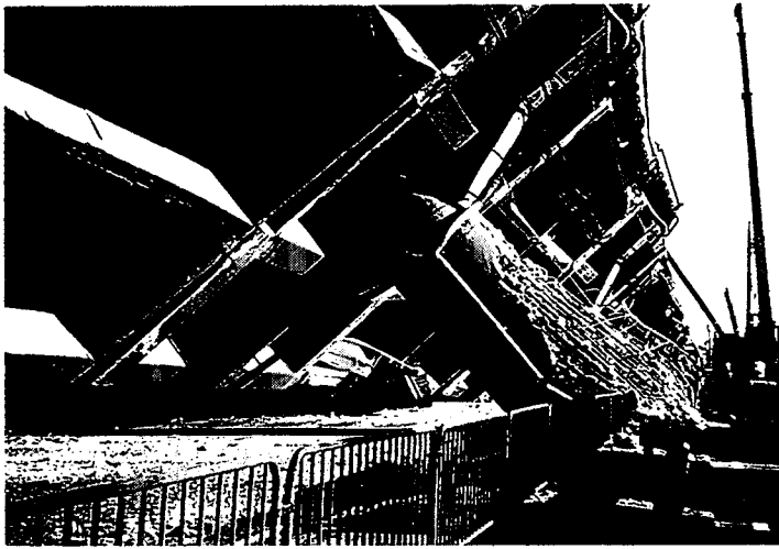
Photo 5 Collapse of pilz-type bridges
