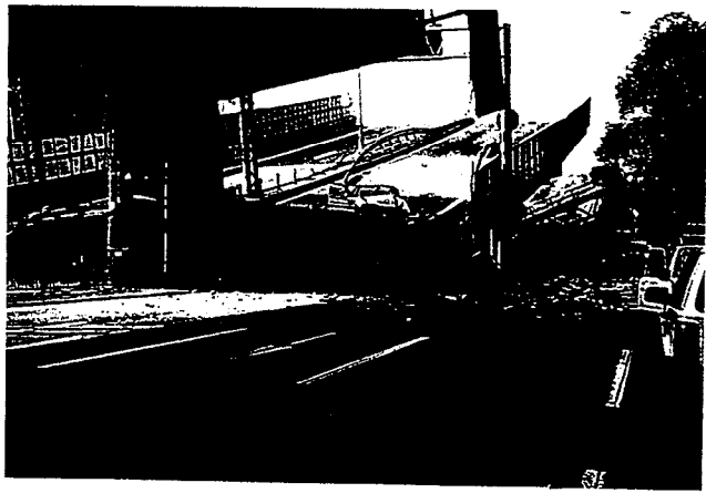
Photo 4 Damage to elevated expressway bridges (Fallen two adjacent simple-beam decks)
