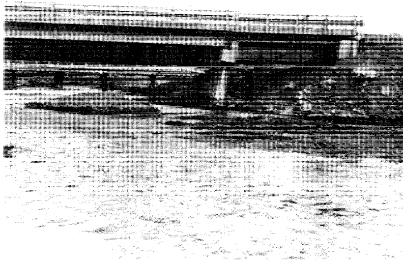
Figure 4. Highway bridge over Resurrection River that was compressed by lateral spreading during the 1964 Alaska earthquake. The compression thrust the deck into and fractured the abutment wall while ground displacement carried the adjacent pier streamward, fracturing that element at the ground line (after McCulloch and Bonilla (6)).
