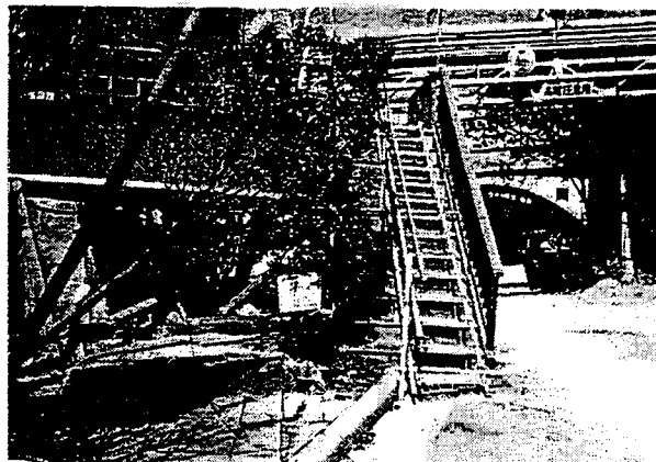
Photo. 6 Separation between stairs of over-canal bridge and its concrete foundation due to ground displacement toward the canal (left) (B in Fig.6)
