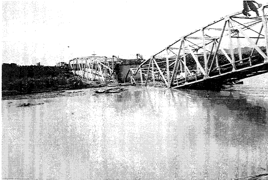
Figure 12. Highway bridge that collapsed into the Rio Estrella during the 1991 Costa Rica earthquake (photograph by T.L. Youd).
