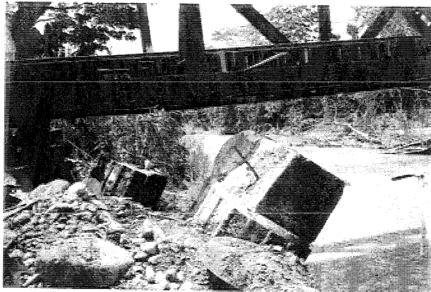
Figure 11. Caissons beneath the Rio Bananito railway bridge that were pushed riverward by lateral ground displacement during the 1991 Costa Rica earthquake (photograph by T.L. Youd).
