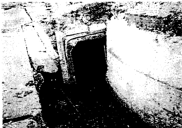
Photo. 7 Floating and separation of concrete conduit due to ground displacement (Courtesy of Mr. K. Takenaka, C in Fig. 6)
