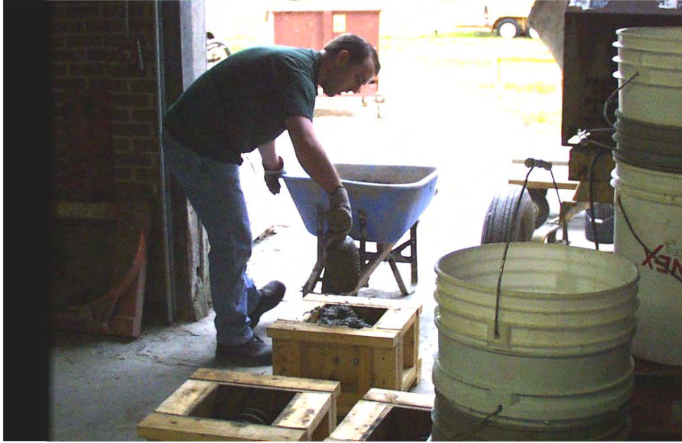
Figure 4.11: Concrete Placement for Pullout Specimens
