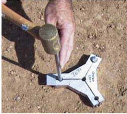
Fig. 5. Driving Spikes Through Template
