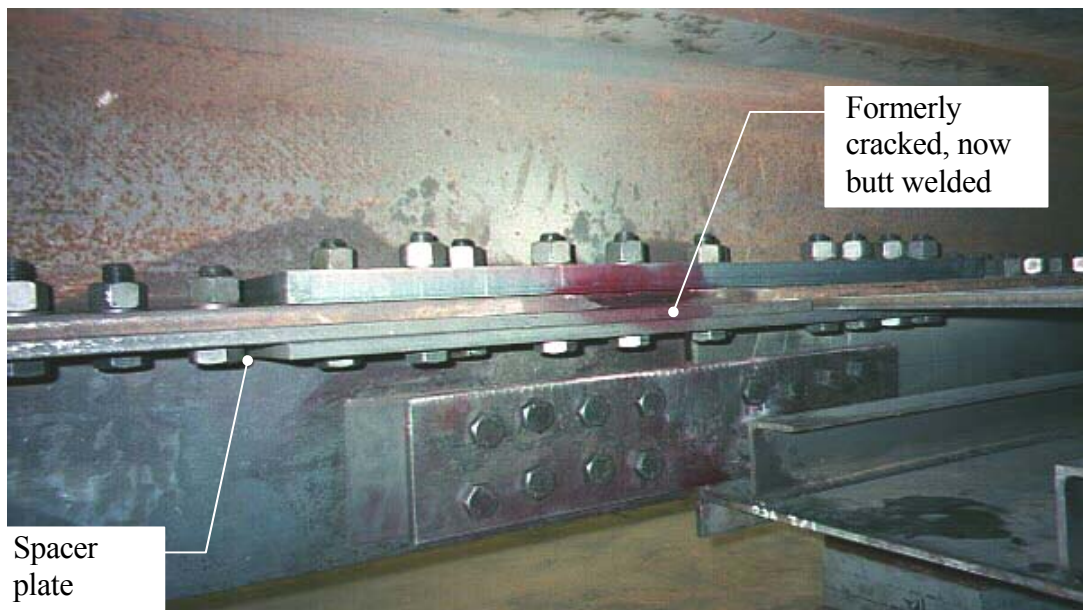
Figure 11-38: Final repair of cracked beam tension flange.
