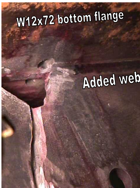
Figure 11-18: Crack faces arc-gouged and crack tips drilled.
