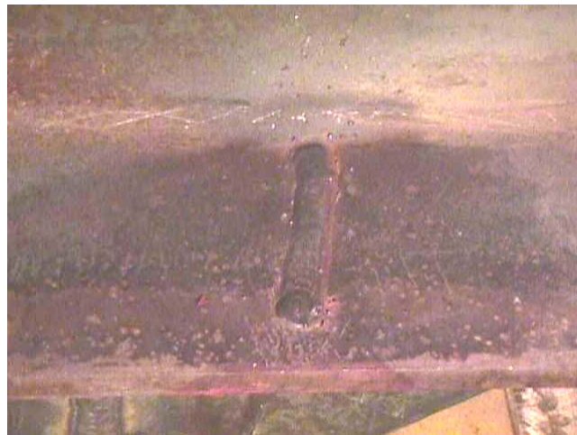
Figure 11-9: Resultant weld between drilled-out crack tips.
