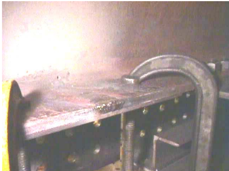
Figure 11-36: Completed butt weld with backing bar in place.
