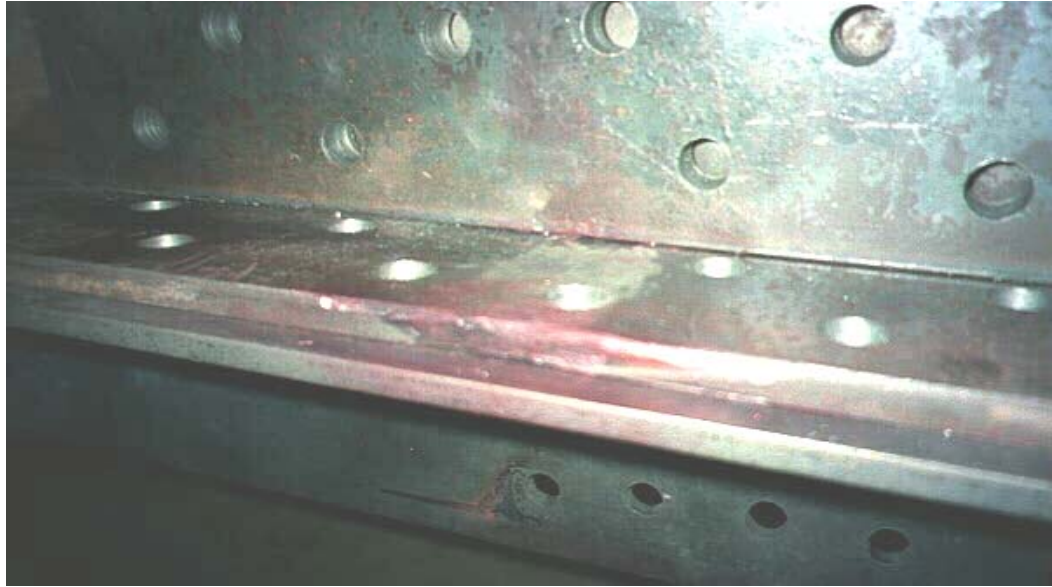
Figure 11-37: Ground butt weld with bolt pattern drilled for adding redundant plates.
