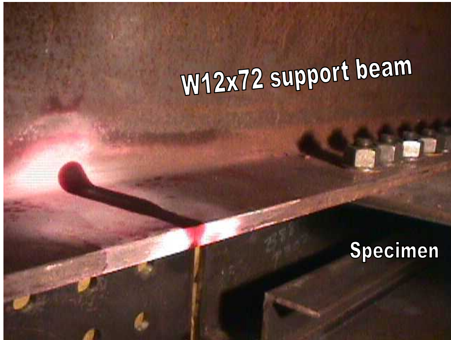
Figure 11-30: Crack in beam tension flange due to abrupt stops in loading.
