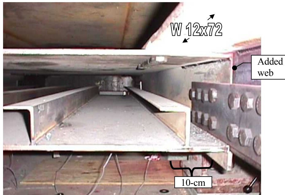
Figure 11-24: Tight clearances for bolting splice plates.
