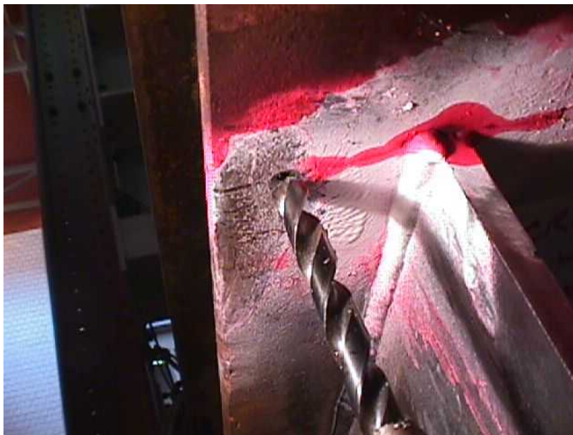
Figure 11-6: Drilling out the crack tips.
