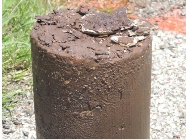
Figure 9. Picture of a Base Core for I-40.
