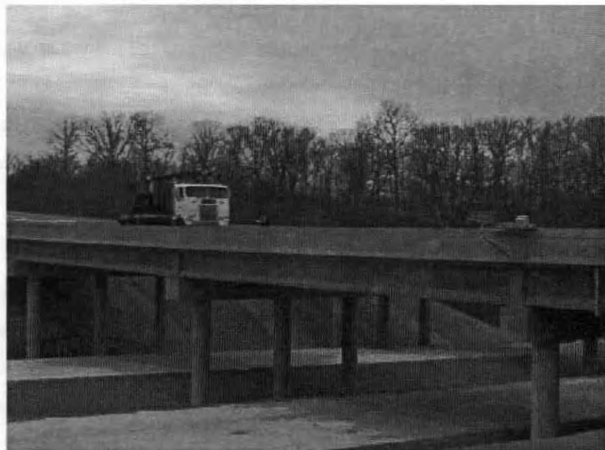
Figure 7.2 Load test in progress
