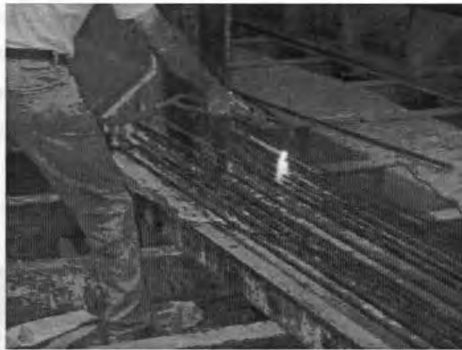
Figure 5.2 Close-up of the process of cutting prestressing strands with a torch
