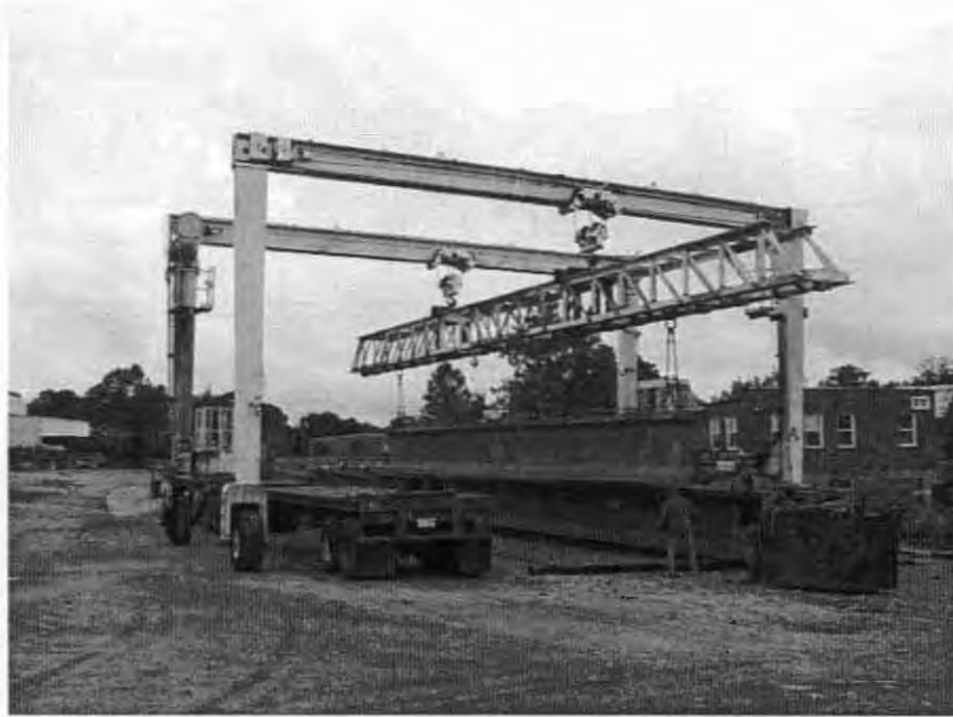
Figure 6.1 Gantry crane used to move girders
