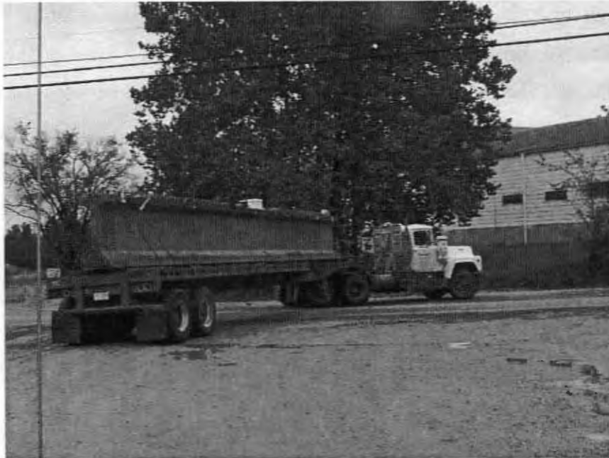
Figure 6.12 Transporting the girder to the bridge site
