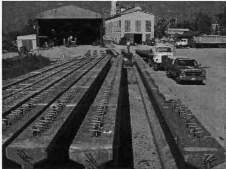
Figure 6.4 Storage of the girders at the precasting yard prior to bridge construction
