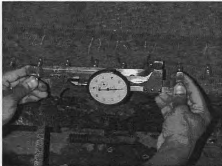
Figure 2.24 Transfer length measurement being made using the Whitmore gage
