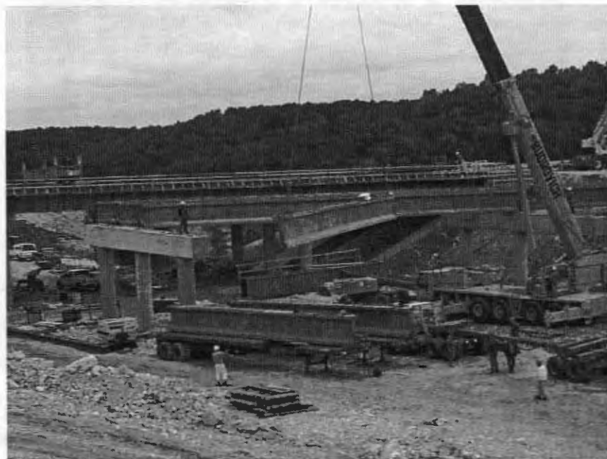
Figure 6.13 Setting the instrumented girders on the bents
