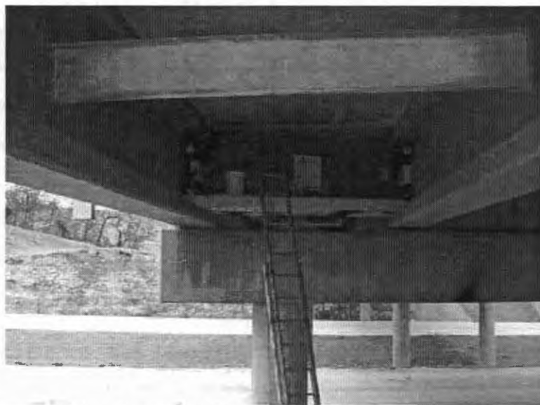
Figure 7.15 Access to the work platform using a 30-ft ladder
