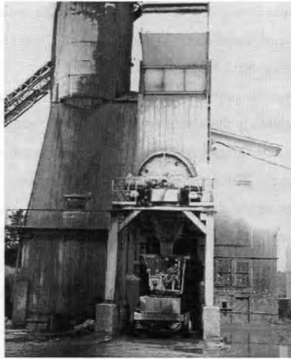
Figure 4.1 The sidewinder being loaded with concrete at the batch plant
