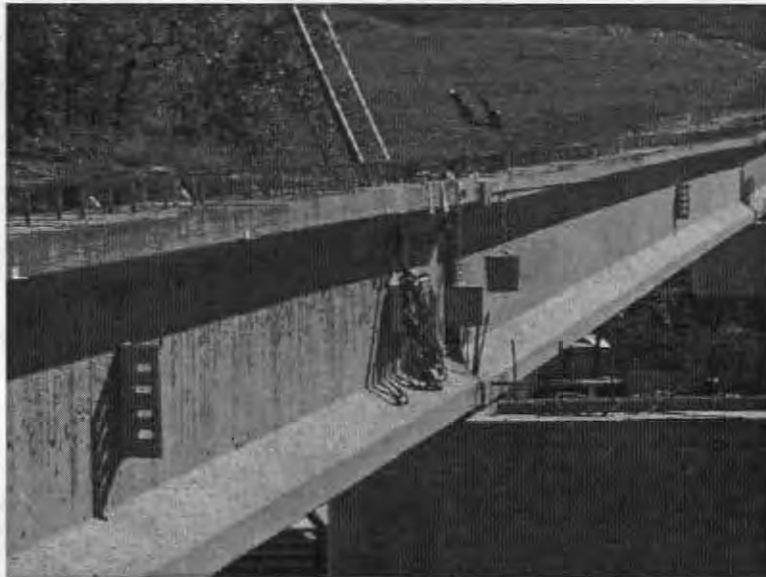
Figure 6.14 Instrumented girders in place on bents
