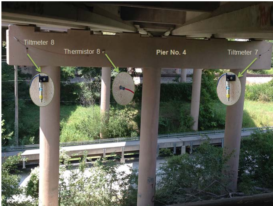
Figure 62 Pier cap instrumentation on Pier No. 4 of the SH-3 north bridge
