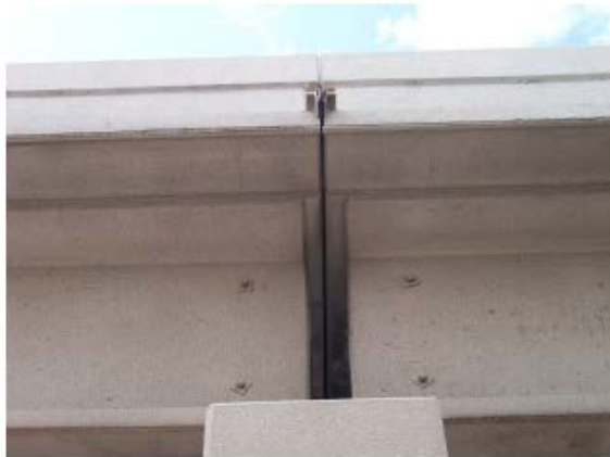
c) Center expansion joint on the South Bridge at 19 th Street
