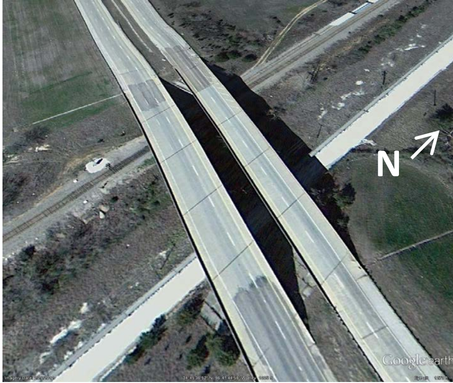
Figure 34. SH-3 bridges over BNSF railroad
