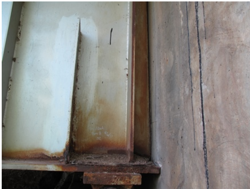
Figure 15. A beam pushing against an abutment backwall on the Shell Creek Bridge
