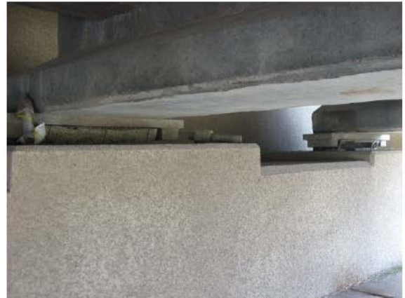
Figure 89. 19 th Street/I-35 Bridge sheared anchor bolts in 2009
