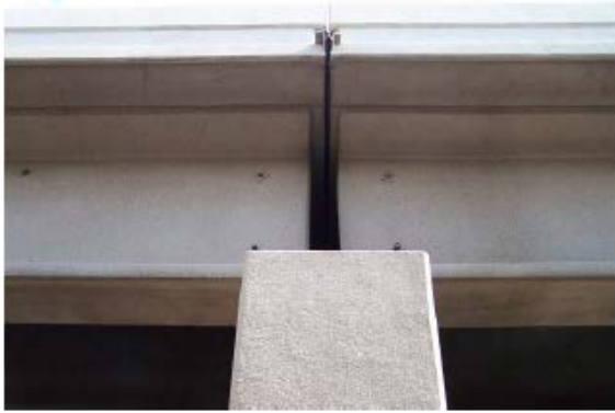
a) Center expansion joint on the North Bridge at 19 th Street
