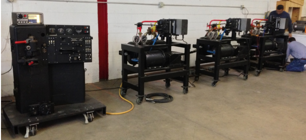
Figure 4-1 – Test Bed for Emulator ECP Assembled in the SA Lab
