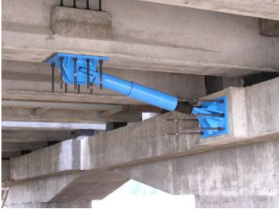
Figure A-1 Longitudinal Damper on Bridges
