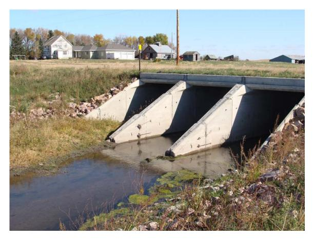
Figure 4.2. Multiple culverts set at same elevation with one culvert filling in with sediment.
