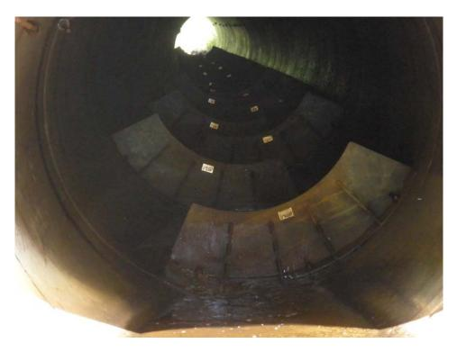
Figure 4.5. Offset baffles retrofit in round concrete culvert. (St. Louis County).
