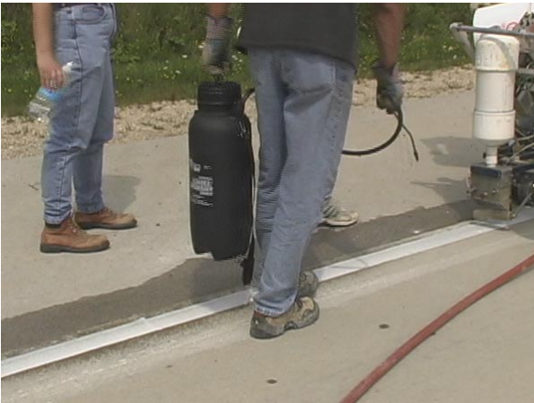
Fig. 6: Spray Cure Application
