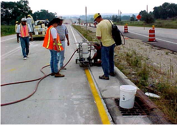
Fig. 8: Lumimark Yellow Edge Line Installation
