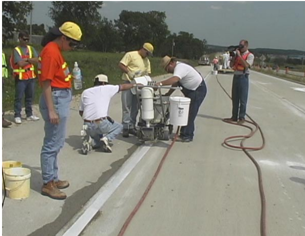
Fig. 5: Placement of White Line
