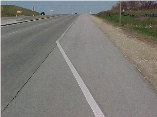
Fig. 10 October 2001 Epoxy Taper Line in Fore Ground Adjoining a White Lumimark Edge Line
