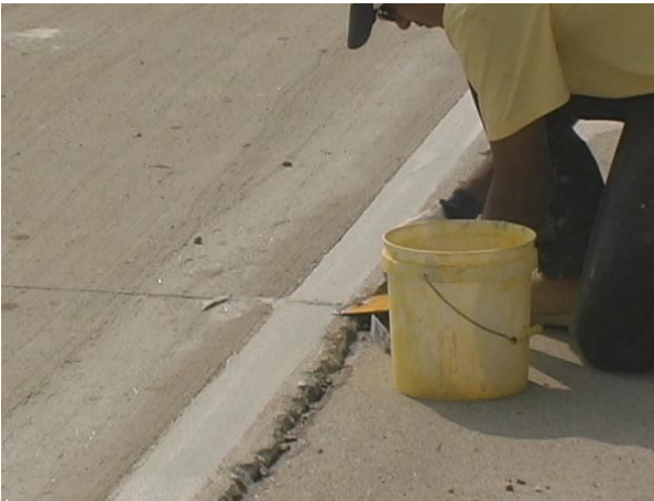
Fig. 7: Cutting of Control Joints
