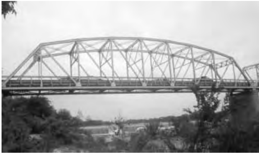
Figure 4.1 Historic Truss Bridge in Llano, TX
