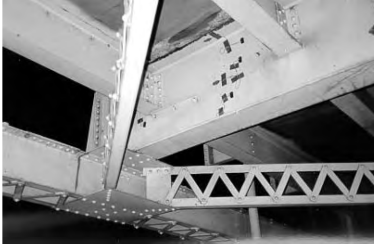
Figure 4.3 Connection of Second Floor Beam to Truss
