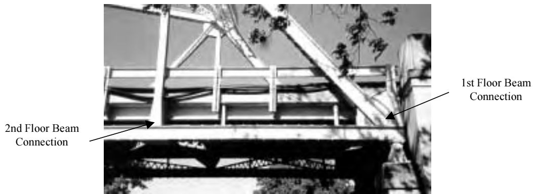
Figure 4.13 Floor Beam to Truss Connections
