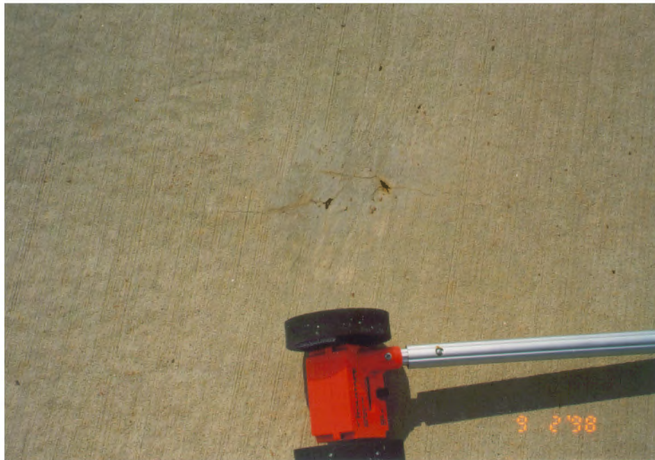
FIGURE B-5. FIBER BALL NO. 1 VISIBLE ON THE SURFACE (SEPT. 1998)
