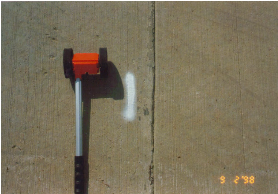
FIGURE B-14. CONSTRUCTION JOINT IN THE PRESTRESSED PAVEMENT (SEPT. 1998)
