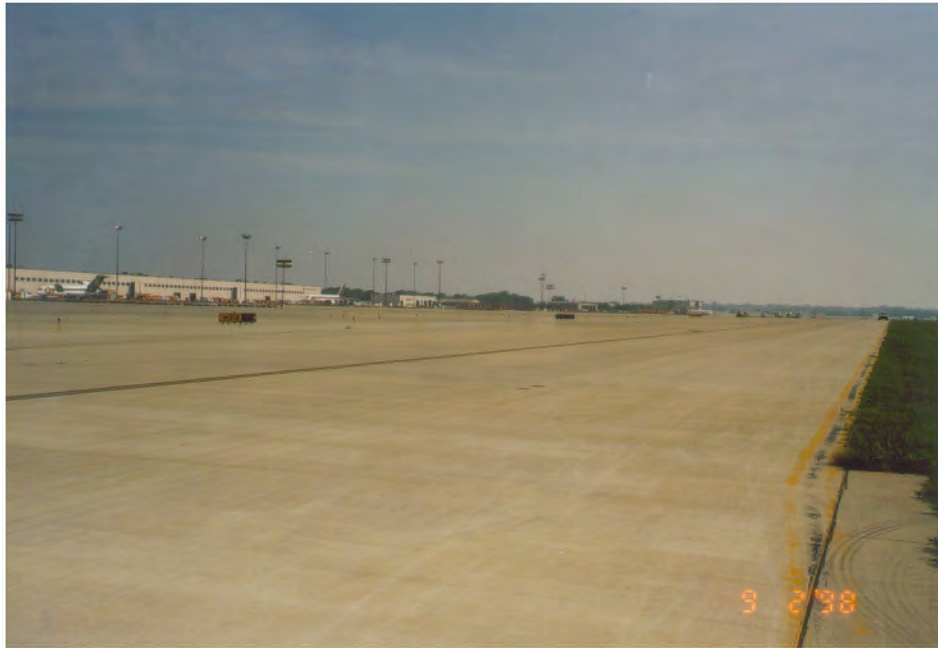
FIGURE B-1. OVERALL VIEW OF PROJECT SITE (SEPT. 1998)
