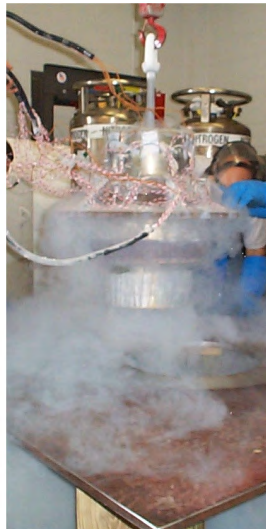
Figure 7.13 Insertion of cooled trunnion-hub into the girder.
