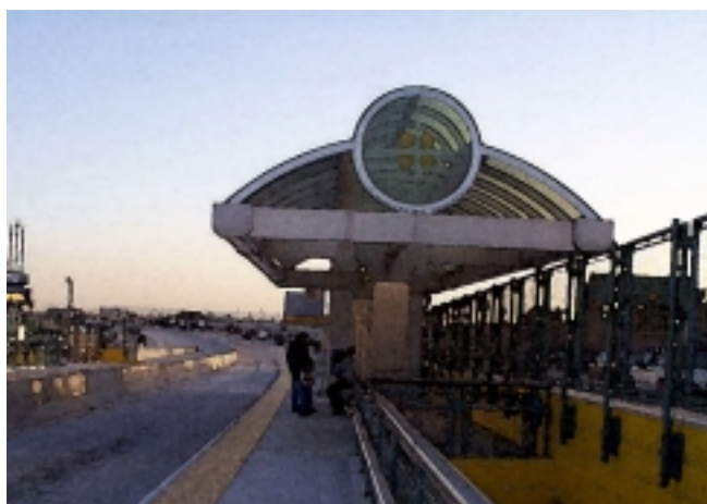
Plate 20: Platform Level Views of the 37 th Street Station
