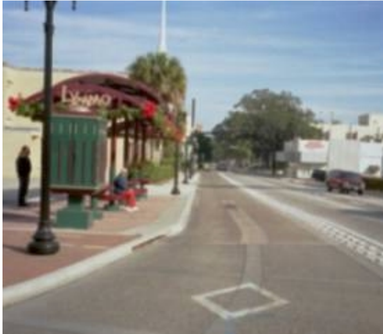
Figure 3.1: Lymmo Right of Way and Station at Turn Around Area
