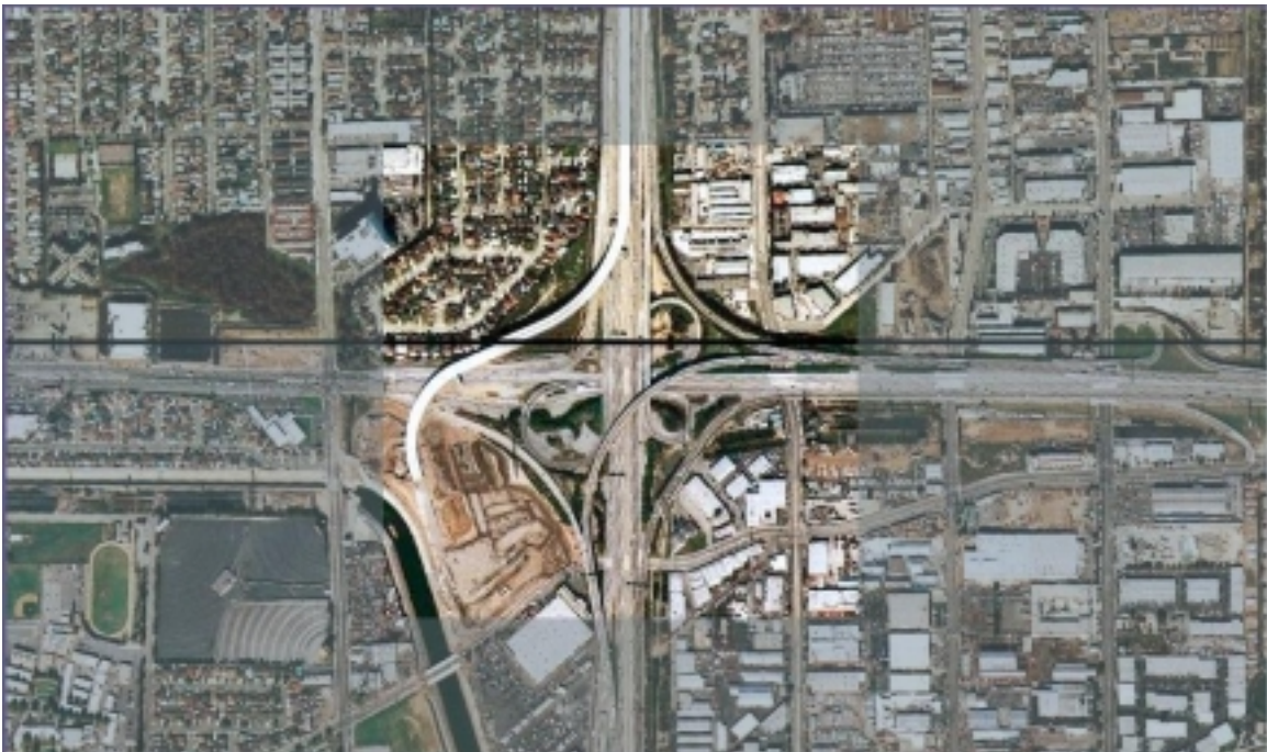
Plate 10: Bus Stop on Harbor Freeway I-110 and Artesia Boulevard
