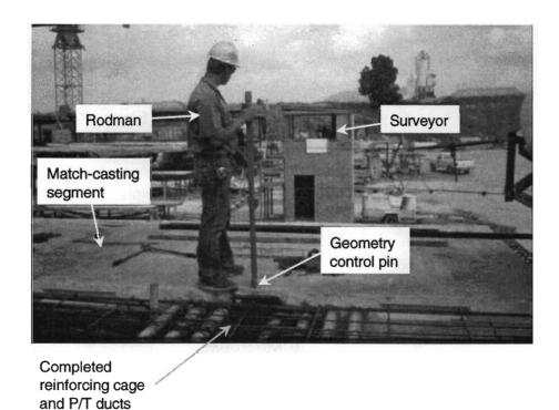
Figure 1.23 Geometry control of the casting machine
