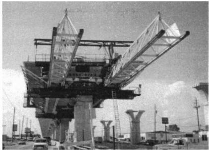
Figure 1.18 Construction of a mainlane girder
