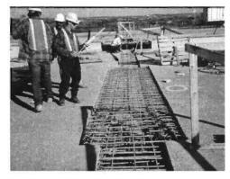
b). Epoxy-coated reinforcing steel in place
