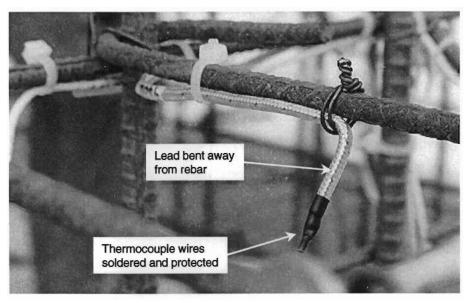
Figure 2.13 Installation of a thermocouple
