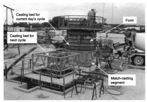
Figure 1.35 Pier segment casting machine
