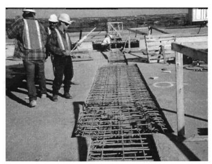
Figure 1.19 Construction of a cast-in-place deck joint
