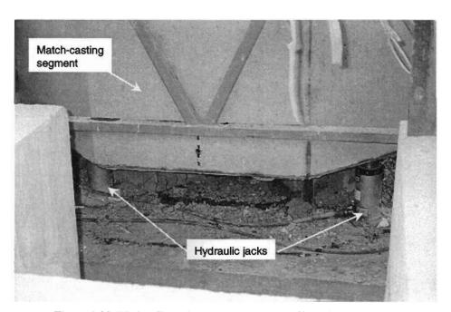
Figure 1.39 Hydraulic jacks used to align the bulkhead pier segment
