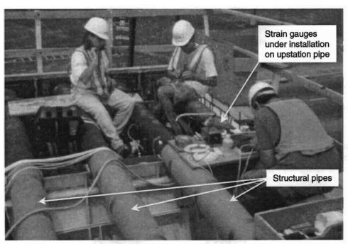
Figure 2.7 "S" series gauges installed on structural pipe
