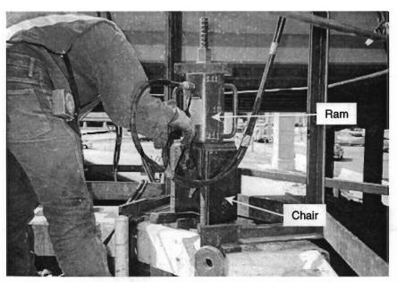
Figure 1.43 Hydraulic ram stressing temporary post-tensioning bars
