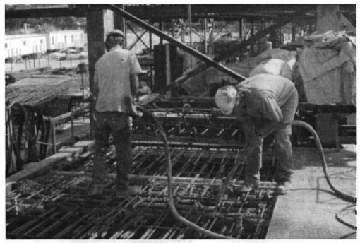
Figure 2.2 Vibrating concrete near instrumentation
