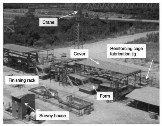
Figure 1.21 Casting machine
