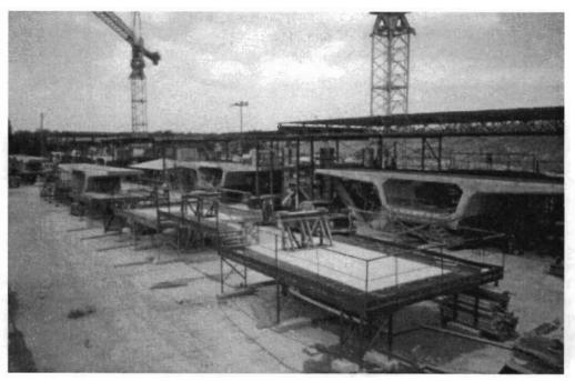
Figure 1.12 Casting machines
