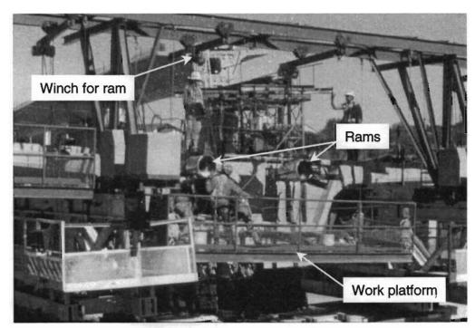
Figure 1.27 Stressing a pair of mainlane girder external tendons
