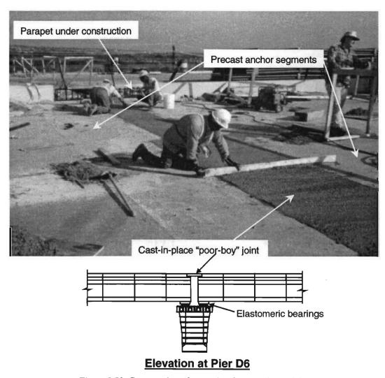
Figure 1.50 Construction of a cast-in-place continuity joint
