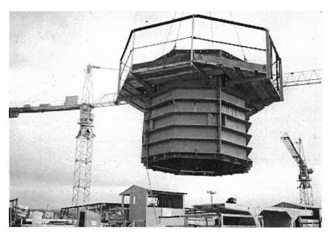
Figure 1.37 Placement of outer pier segment form
