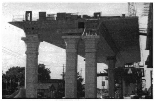
Figure 1.9 Cast-in-place transition spans
