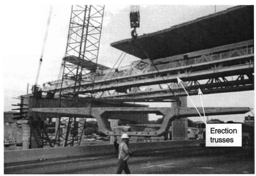
Figure 1.2 Span-by-span construction
