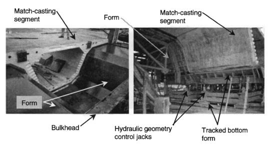
Figure 1.22 Casting machine details
