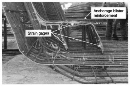
Figure 2.5 "S" series gauges installed on rebar
