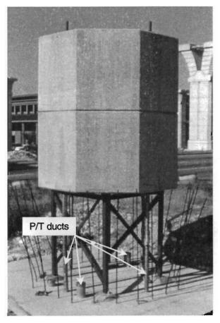
Figure 1.41 Steel support frame for first precast segment
