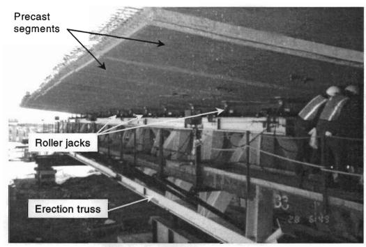
Figure 1.25 Locating segments on the erection trusses
