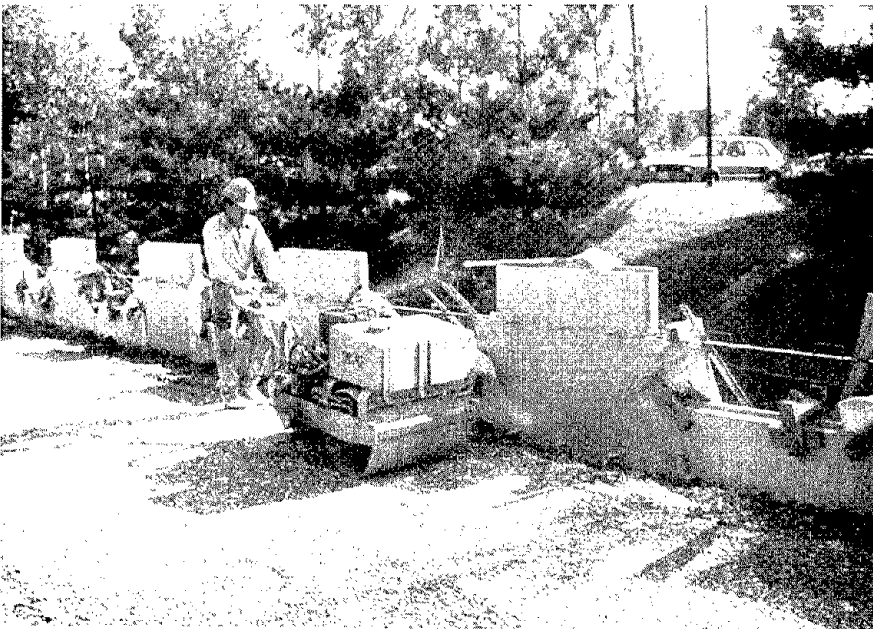
Figure 80. Compaction equipment showing a) large equipment permitted away from face and b) lightweight equipment within 1 m of the face.
