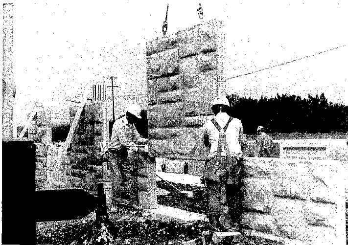
Figure 11. Erection of precast panels.
