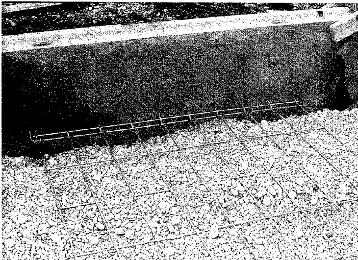
Figure 12. Fill spreading and reinforcement connection.
