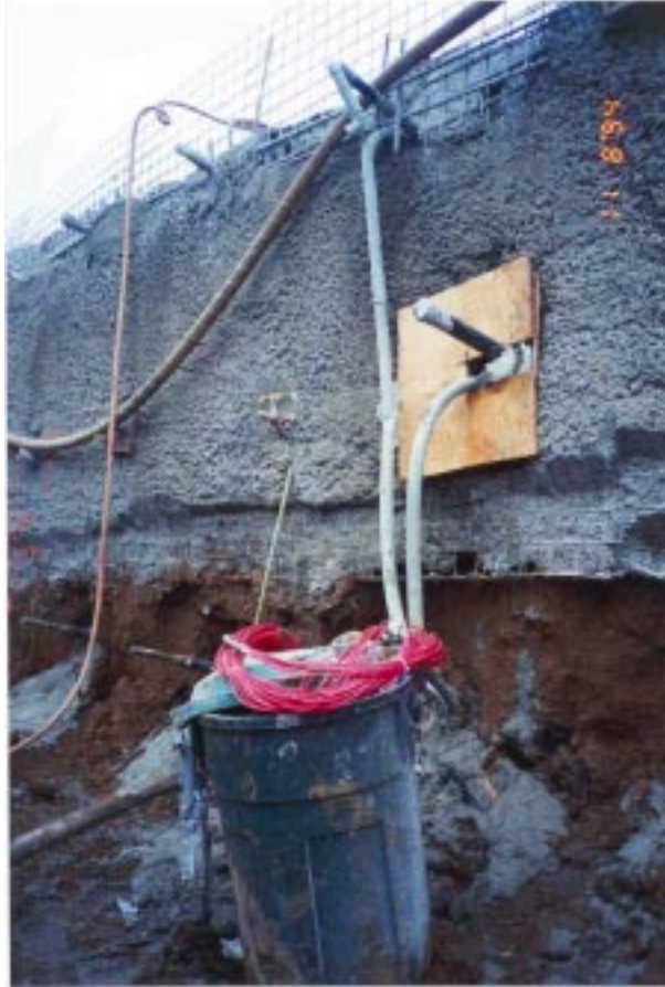
Figure 5.5: Installed soil nail
