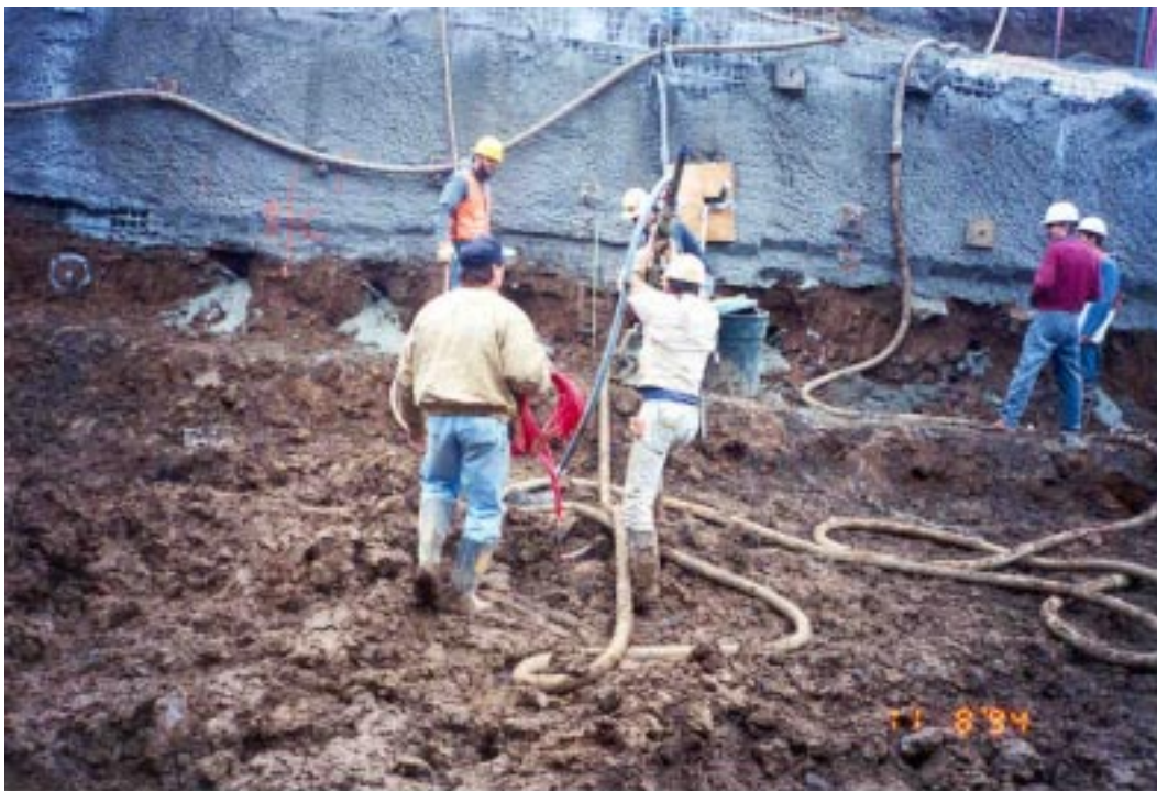
Figure 5.4: Instrumented soil nail installation
