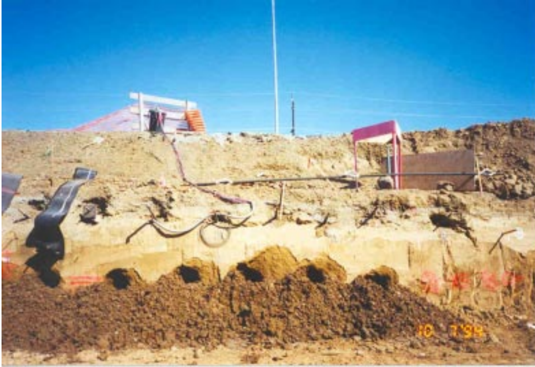
Figure 5.3: Drilled nail holes
