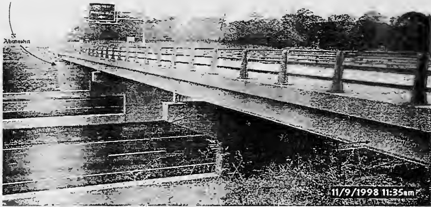
Figure 6.1 Image of A Typical Highway Steel Bridge
