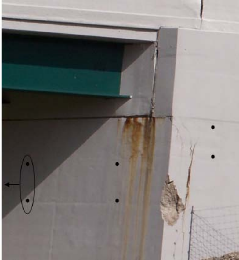
Figure 27: Tilt Reference Stations (East Bound Bridge)
