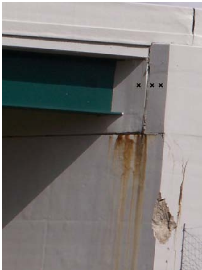
Figure 25: Target Location (East Bound Bridge)
