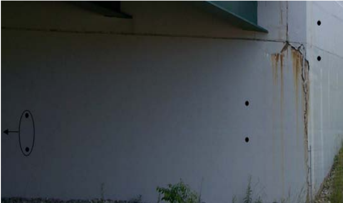
Figure 28: Tilt Reference Stations (West Bound Bridge)
