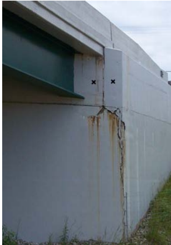
Figure 26: Target Location (West Bound Bridge)
