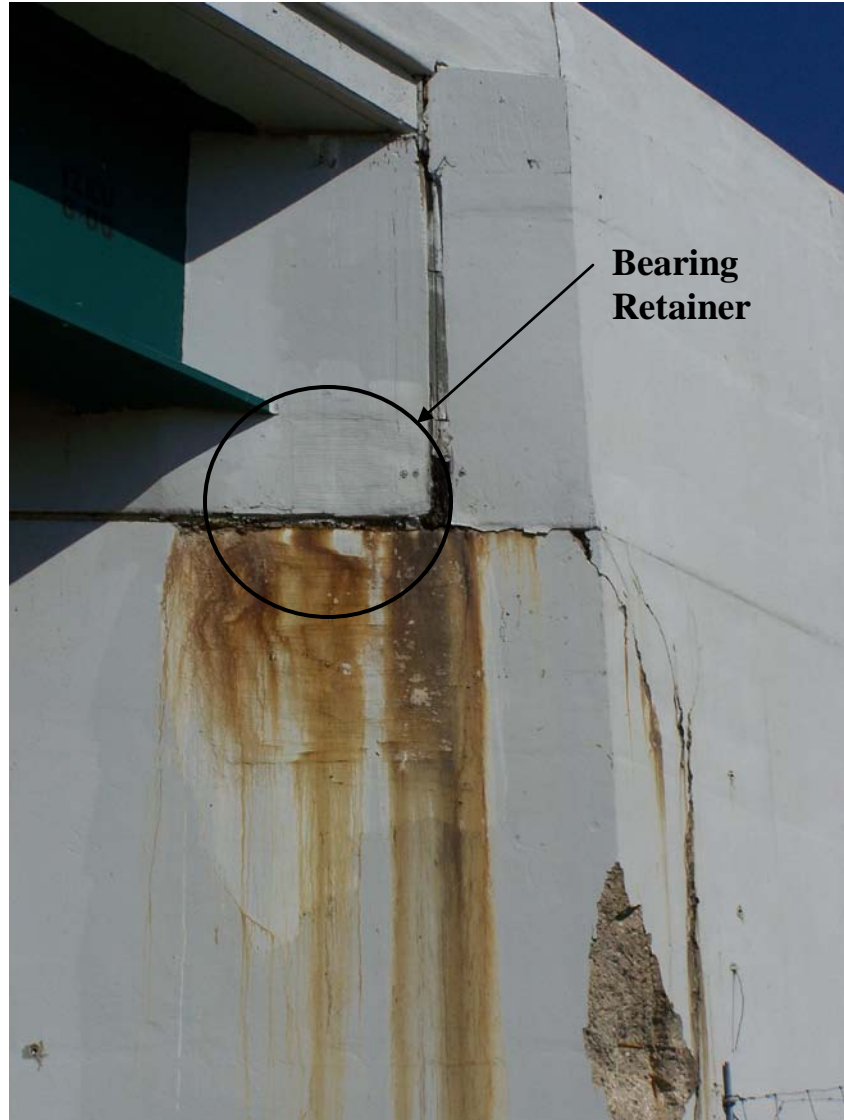
Figure 54: Bearing Retainer (MUS-16-0261)
