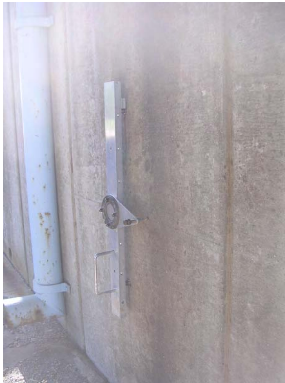
Figure 31: Reference Plate on Wall Abutment (Masada, 2007)
