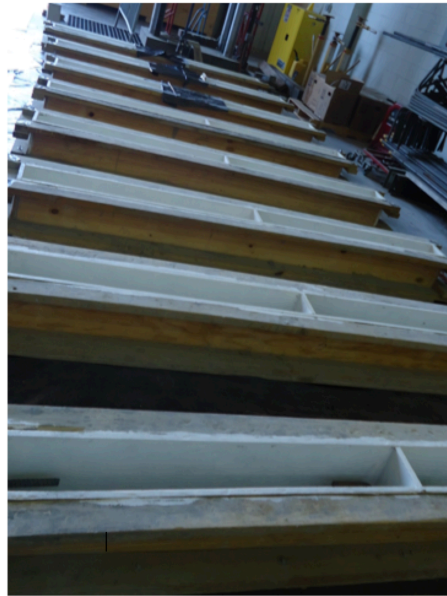
Figure 29. Concrete beam formwork.
