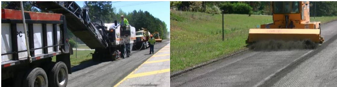
Figure 3-12 Removal of the Existing Pavement Surface
