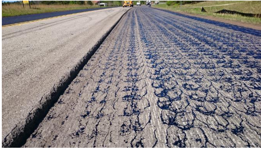
Figure 3-13 Application of Asphalt
