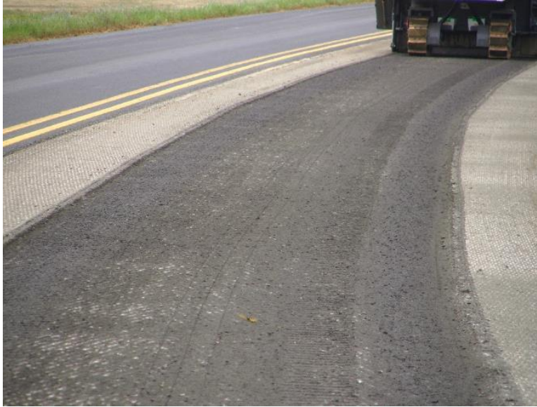
Figure 3-7 Removal of a Thin Layer of Pavement
