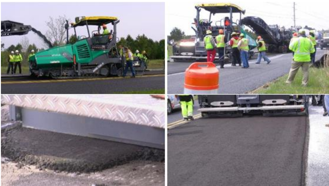
Figure 3-10 Compaction of Recycled Material
