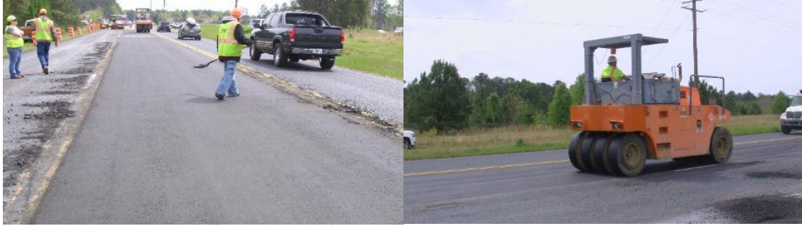
Figure 3-11 Compaction of Recycled Material
