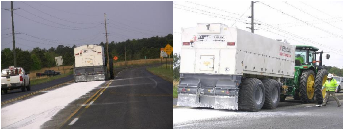
Figure 3-8 Application of Lime on the Milled Surface
