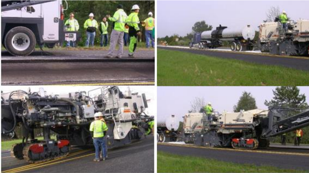
Figure 3-9 Mixture of Pavement and Additives
