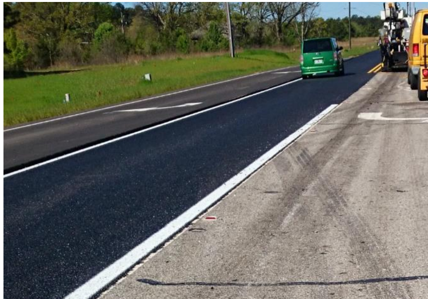
Figure 3-15 Application of 1" OGI
