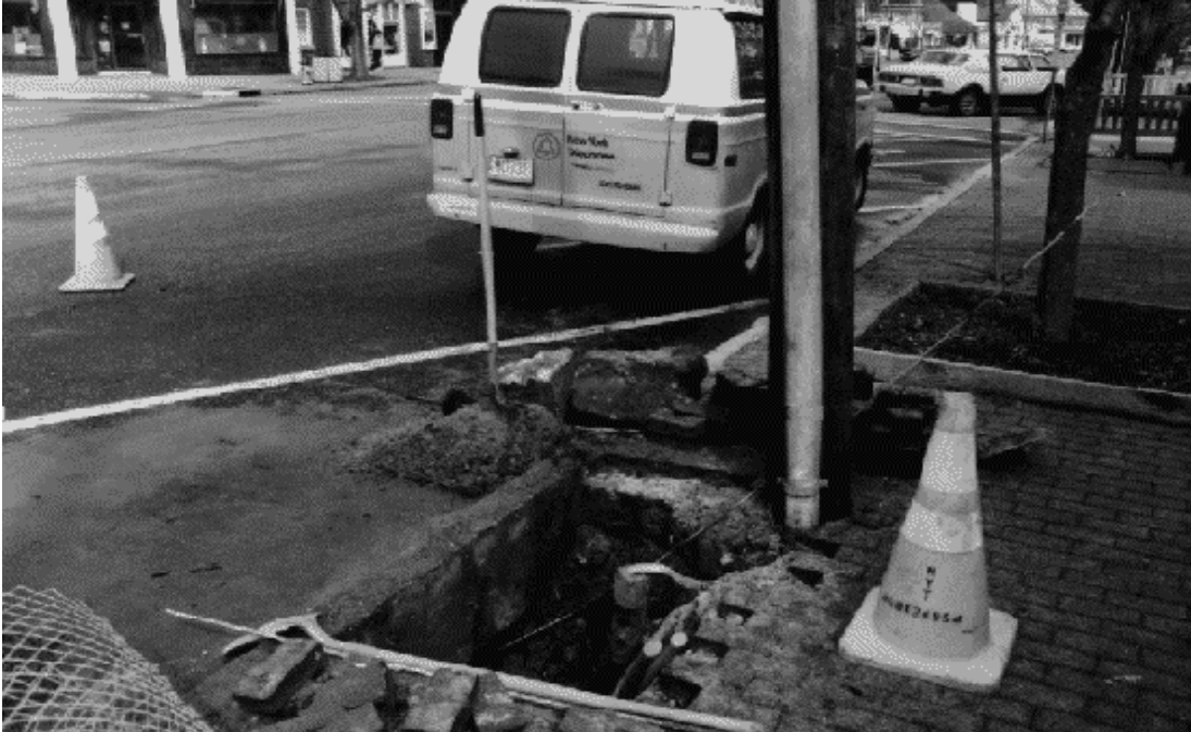
Figure 9-1. Installing communications cable.
