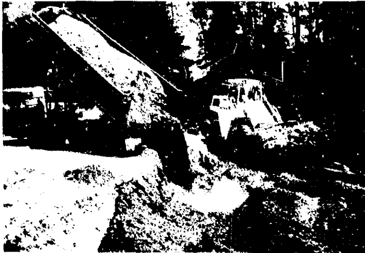
Figure 8 - As the stockpiled material was being placed additional trucks end-dumped the sawdust into the excavated site.
