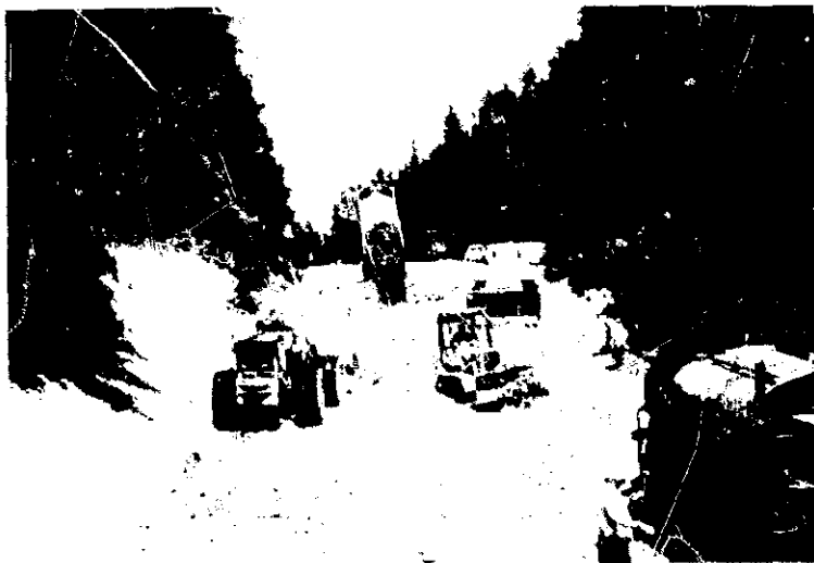
Figure 12 - Sawdust was placed in 1-foot lifts and was compacted with construction equipment in a predetermined pattern.
