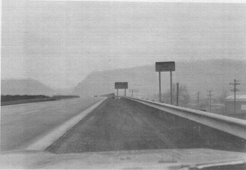
Figure H-10. Signs 5 and 6 and View of Bridge at Station 173
