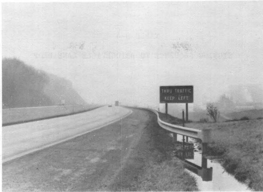
Figure H-8. Sign 2 and View Looking South at Station 202
