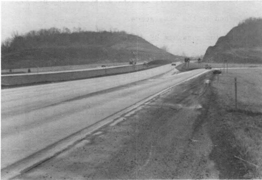
Figure H-12. Sign 8 and Exit Lane Drop at Station 155
