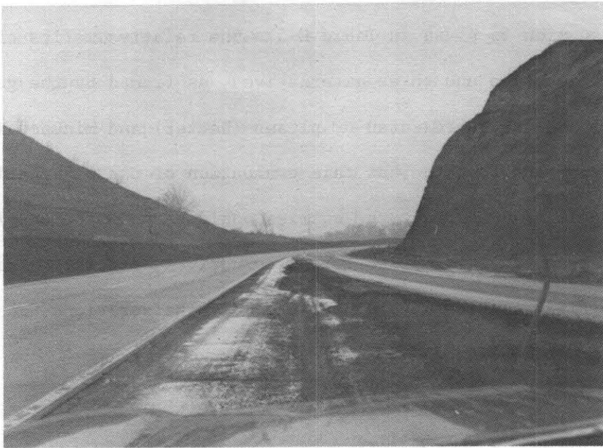
Figure H-14. Bridgeville Entrance Terminal at Station 142
