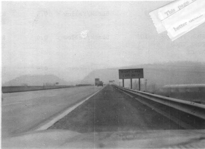
Figure H-9. Sign 4 and View Looking South at Station 178
