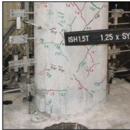
DS-2: first spalling and shear cracks
