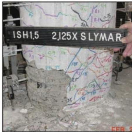
DS-4: lateral and longitudinal bars visible
