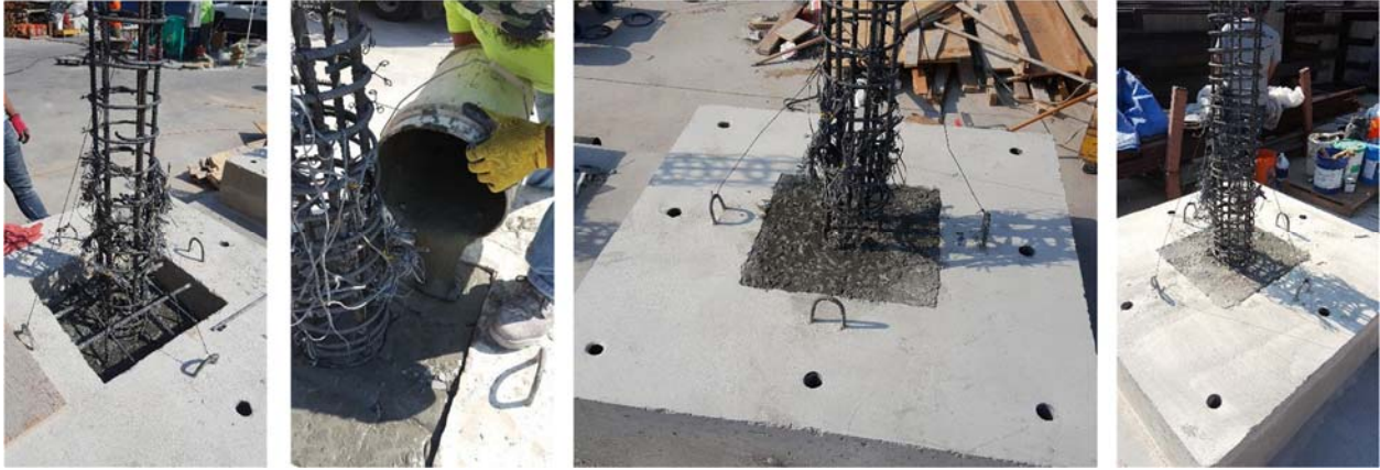
Figure 4-3 Casting of UHPC footing.
