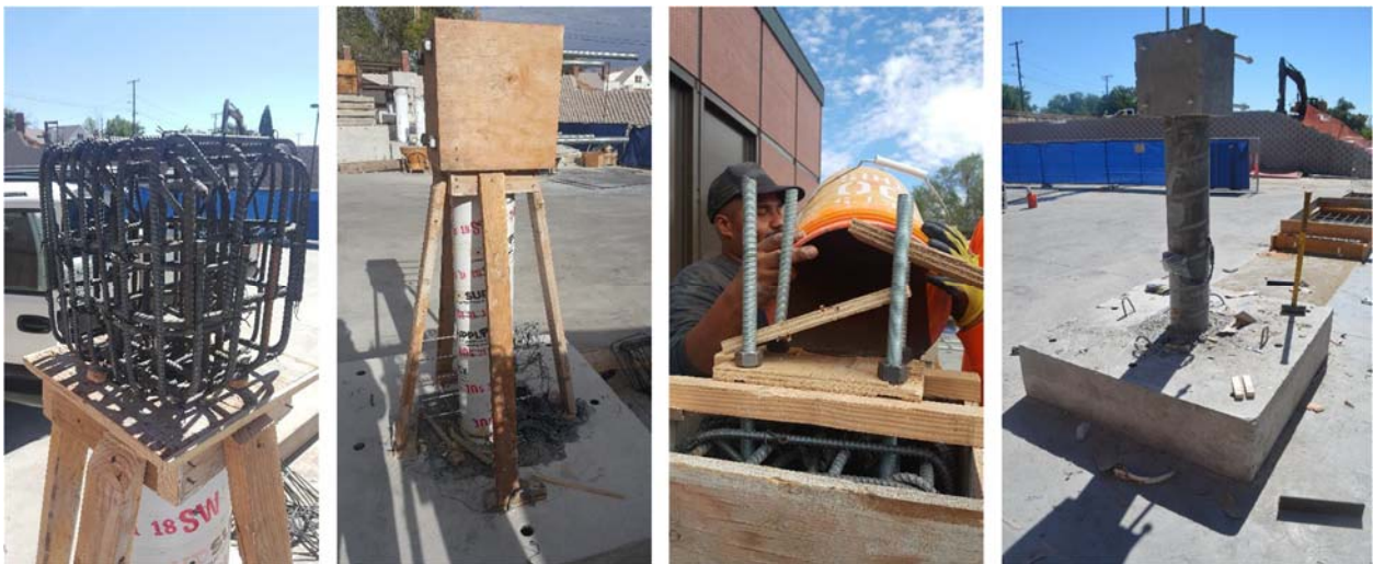
Figure 4-5 Casting of UHPC column head.
