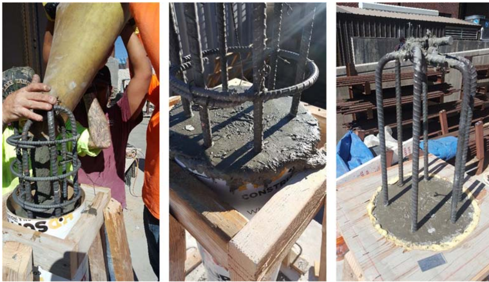
Figure 4-4 Casting of UHPC column.
