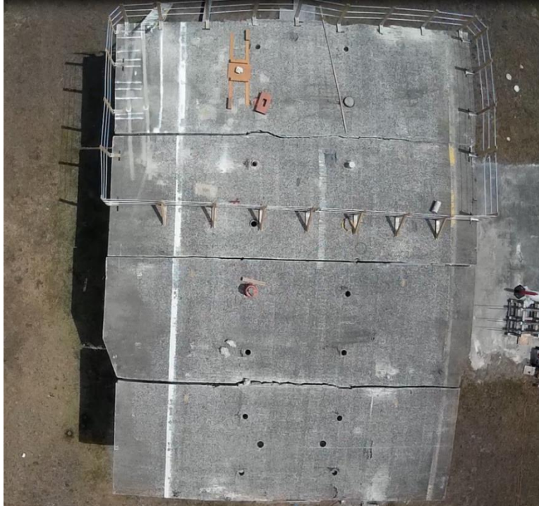
Figure 14: Aerial view of the whole bridge segment.
