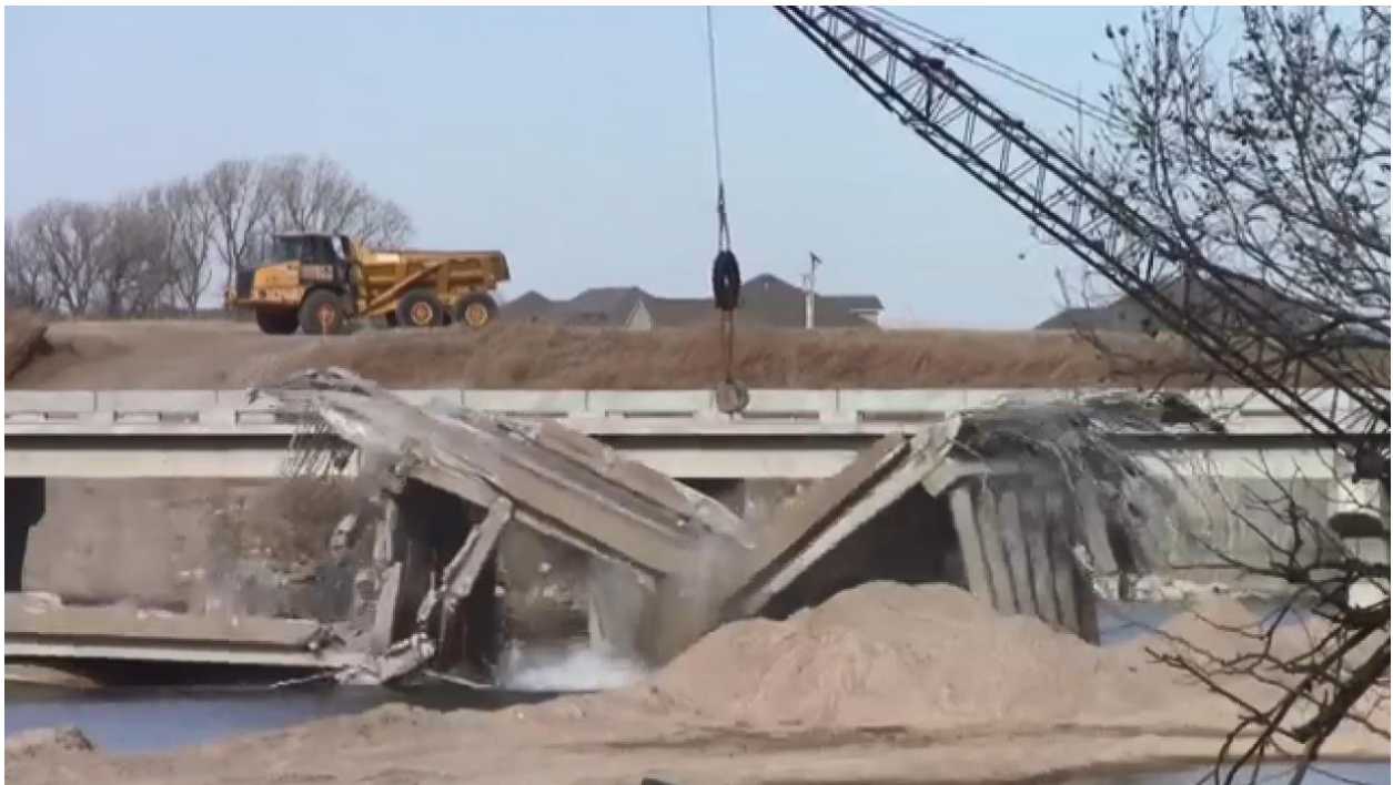
Figure 61. The one last remaining deck of I-235 Bridge demolished by the wrecking ball
