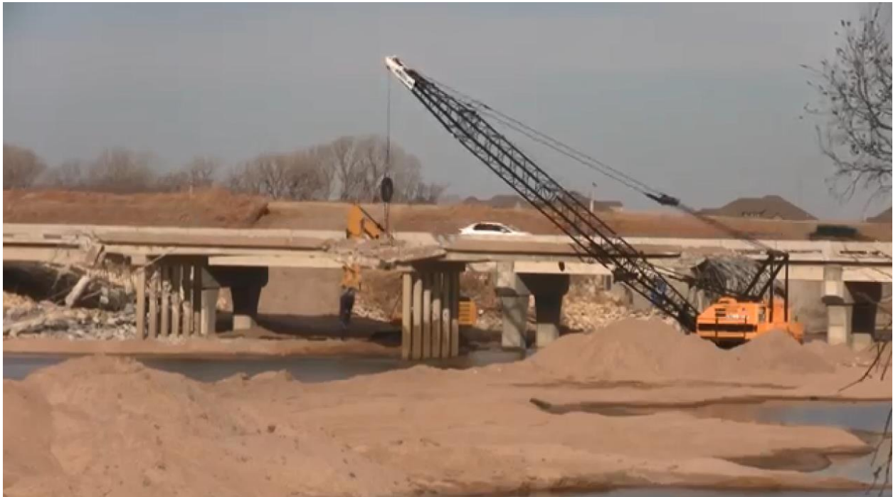
Figure 64. I-235 Bridge with two spans about to be demolished by dropping a wrecking ball
