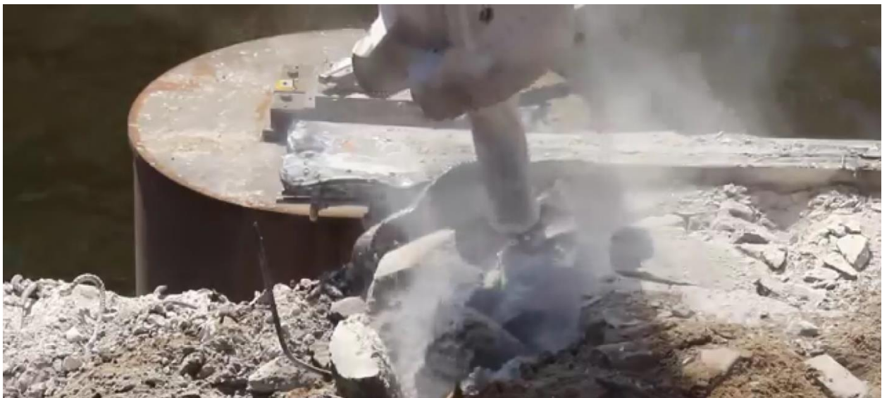
Figure 72. Dismantling demolition using a jackhammer
