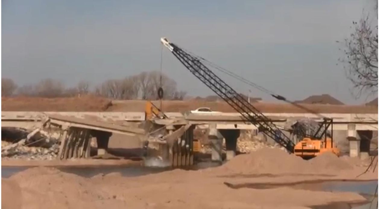
Figure 65. The one of the remaining decks of I-235 Bridge demolished by the wrecking ball
