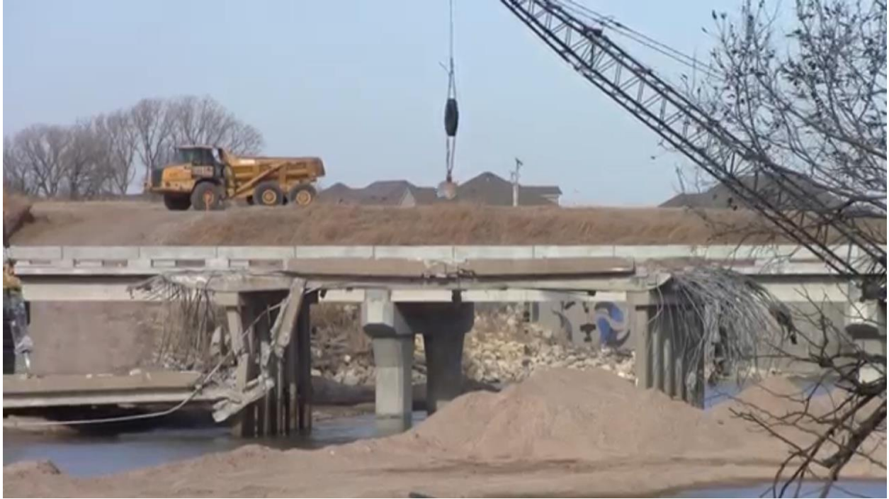
Figure 60. I-235 Bridge with a span about to be demolished by dropping a wrecking ball
