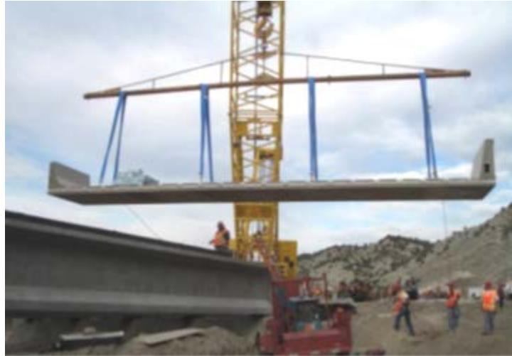
Figure 6.11: Precast Concrete Deck Panel with Integral Barrier [32]
