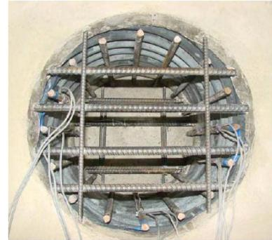
(b) Cap Beam Bar Cage (Left) and Pocket Inside View (Right) for CPF
