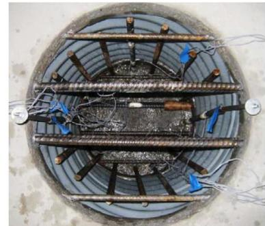
(c) Cap Beam Bar Cage (Left) and Pocket Inside View (Right) for CPLD
