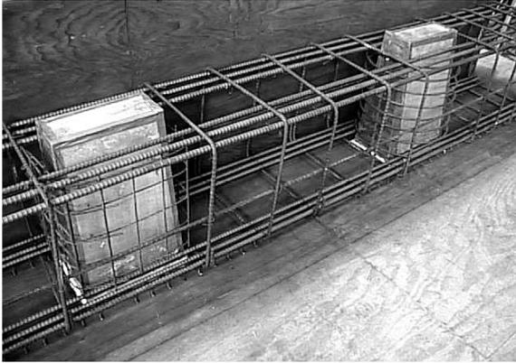
(a) Rebar Cage for Single-Line Pocket
