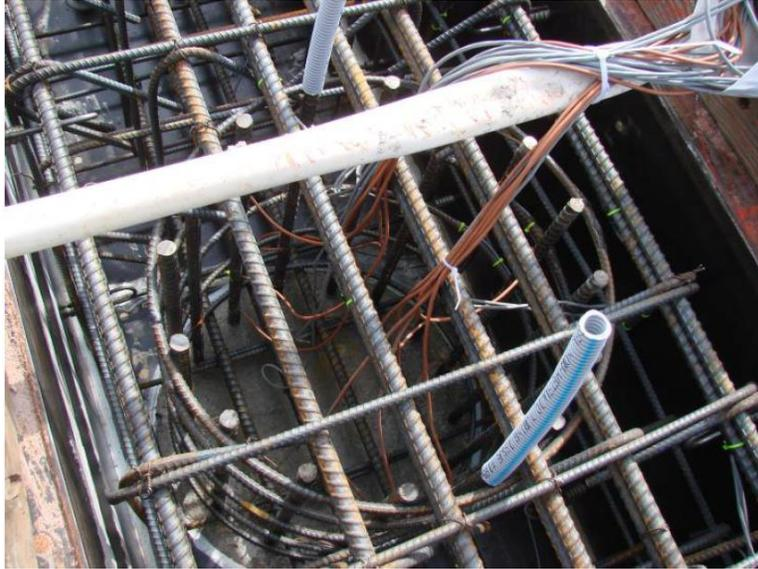
(a) Column to Cap Beam Connection for CIP
