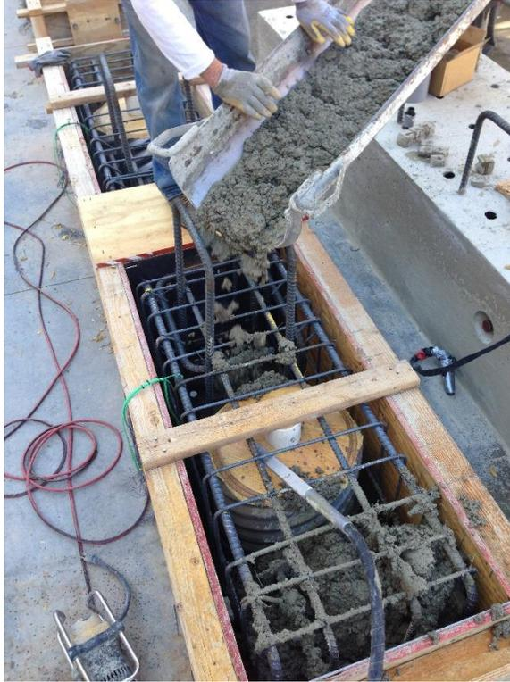
**Figure 1-10. Cap Beam Pocket Connections (Mehraein and Saiidi, 2014)**
