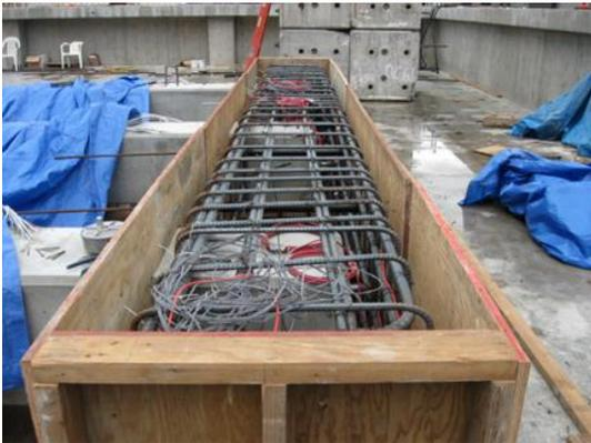
(b) Pile Embedded into Bent Cap (Cukrov and Sanders, 2012)
