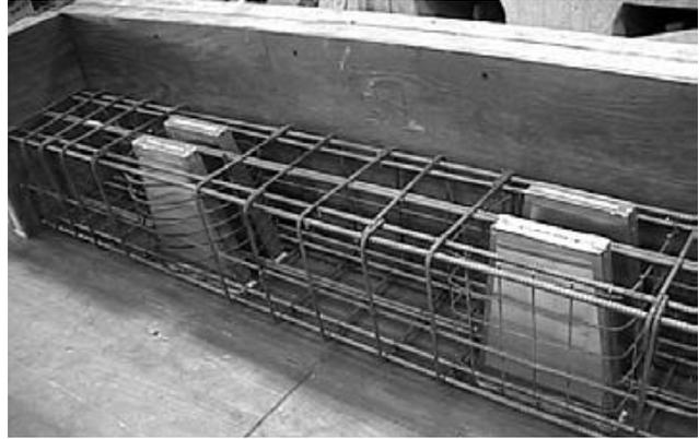
(b) Rebar Cage for Double-Line Pocket
