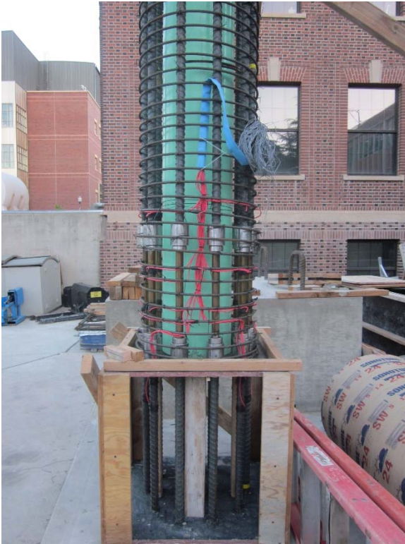
(a) SMA-Steel Bar Cage
