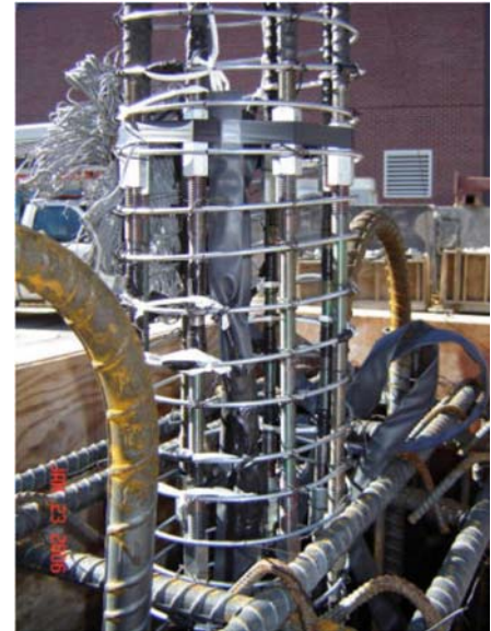
(b) Cage w/ Threaded Couplers
