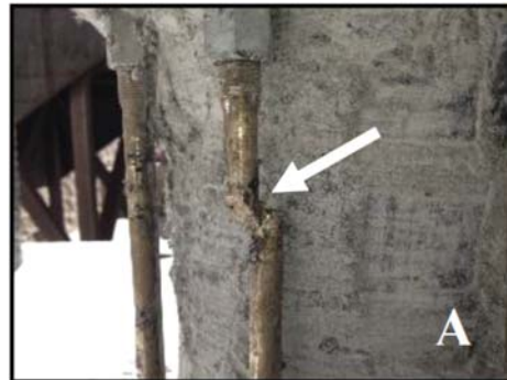
Figure 1-53. Cast-in-Place Column with Threaded Couplers (Varela and Saiidi, 2014)
