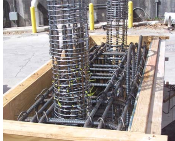
(b) Shear Screw Couplers
