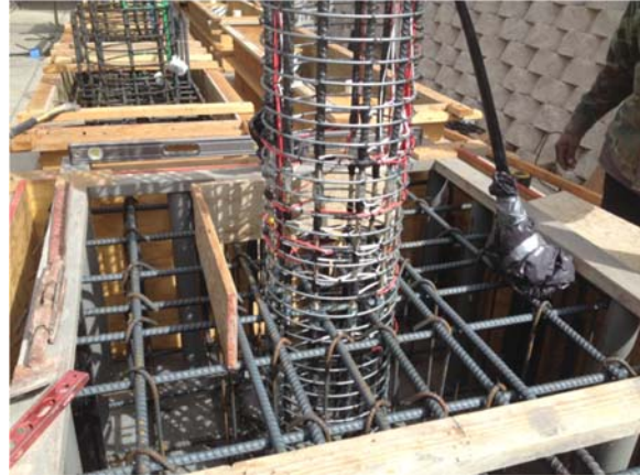
(b) Cage w/ Threaded Couplers
