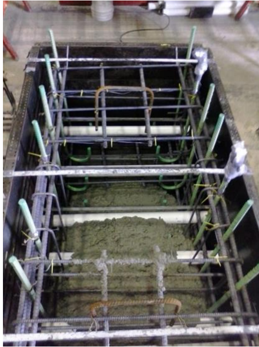
Figure 23. Pile cap reinforcing bar, formwork, and pour
