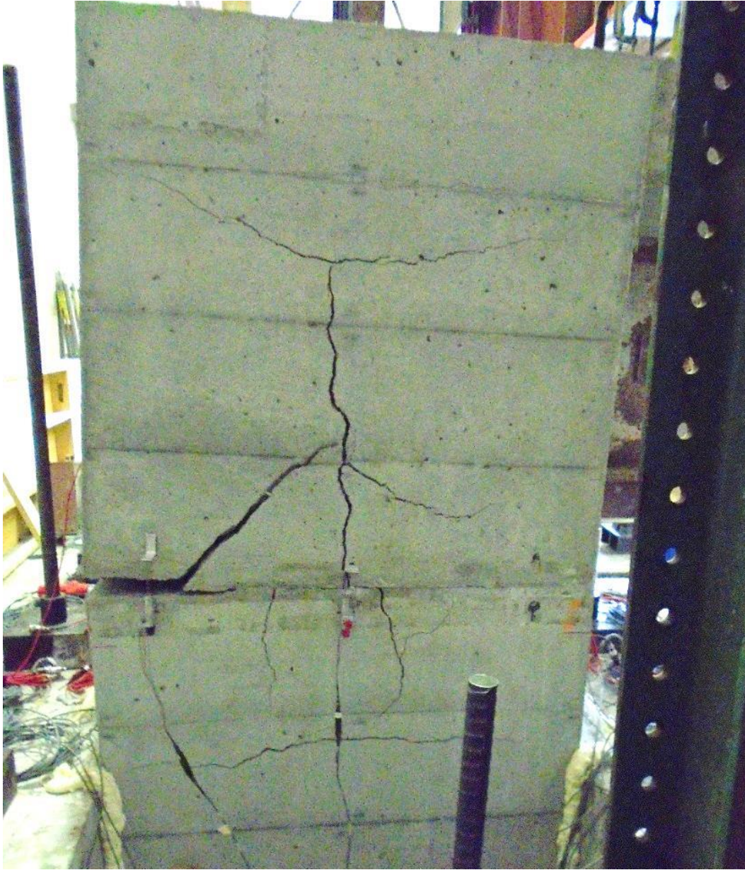
Figure 77. Pile coupler damaged east side
