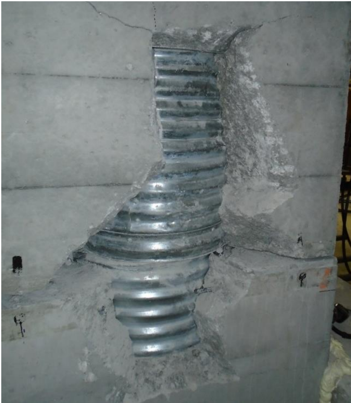
Figure 78. Pile coupler deconstruction
