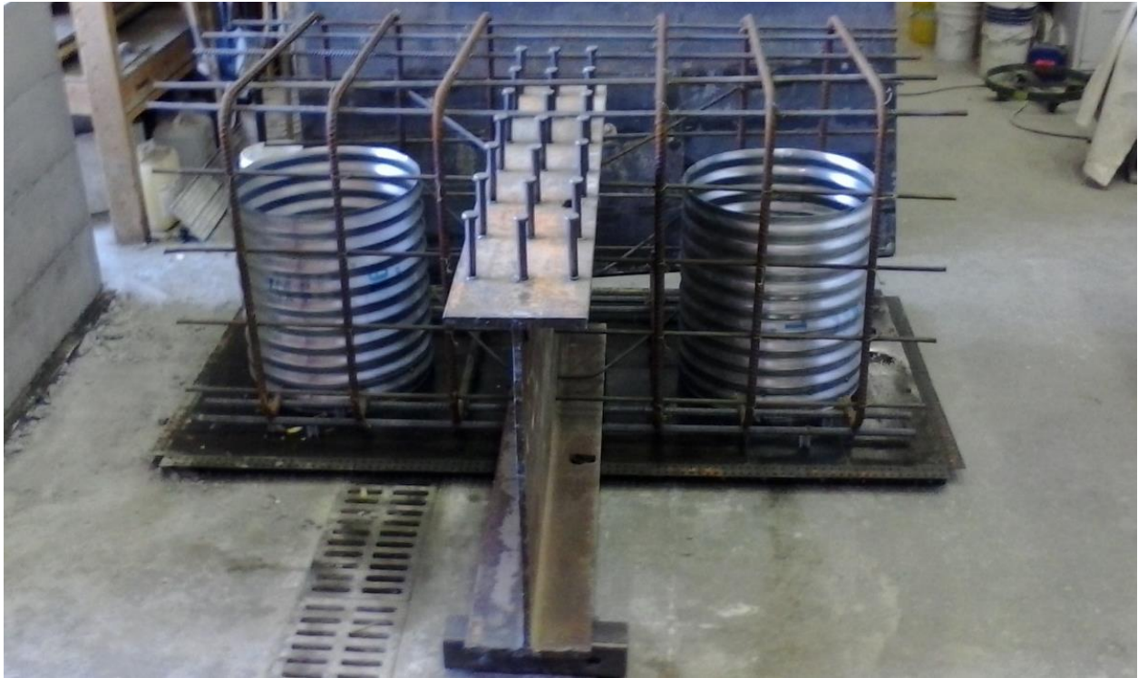
Figure 43. Integral diaphragm reinforcing bar cage
