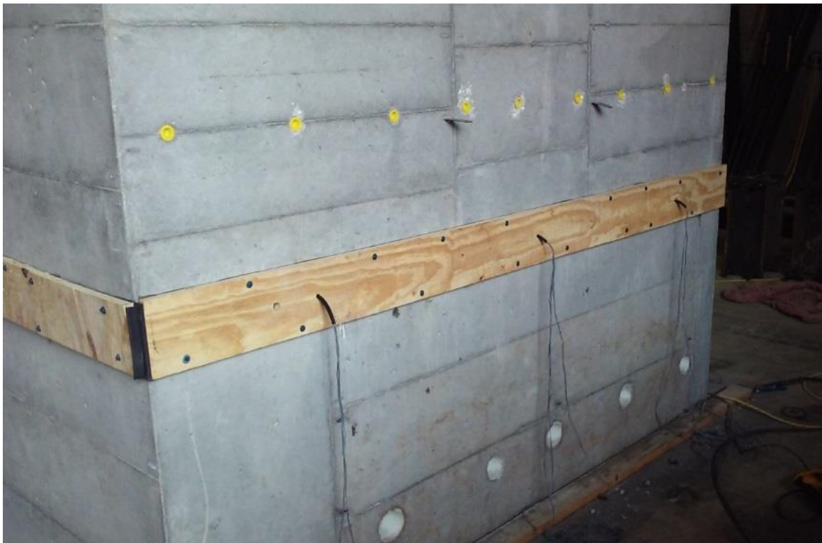
Figure 33. Grout bed formwork
