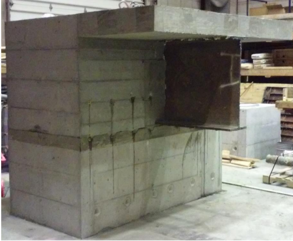
Figure 35. Completed grout bed and coupler grouting
