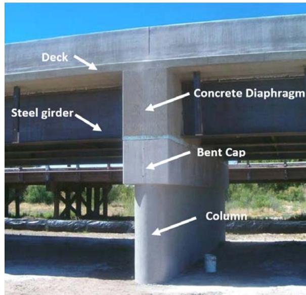
Figure 2-3 Different components of SDCL bridge system.
