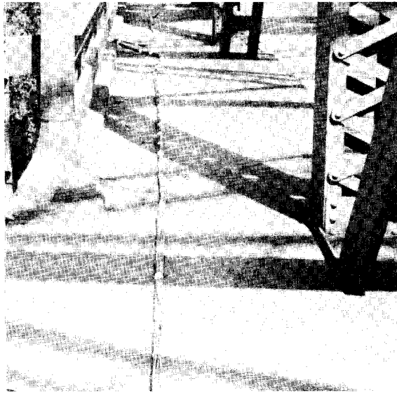
Figure 79. Cable being prepared to be lowered over bridge deck.
