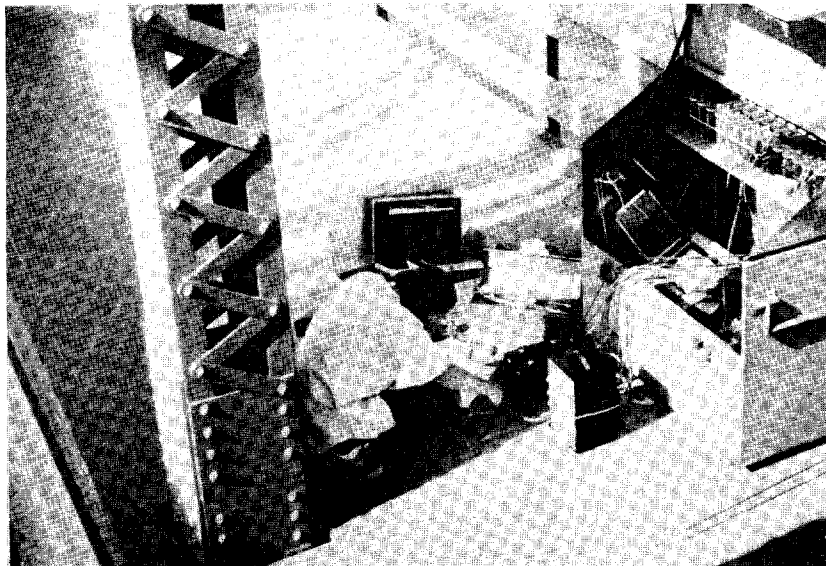
Figure 84. Instrumentation housing on sidewalk over instrumented Pier 6.
