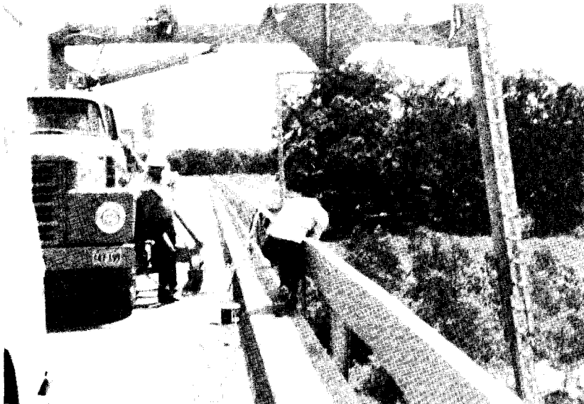
Figure 129. Snooper being used to attach cable to rear of pier. (Snooper furnished by Texas Highway Department)
