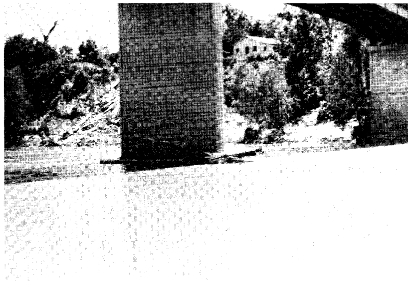
Figure 120. U. S. Highway 59 West Bridge over the Brazos River at Richmond, Texas.
