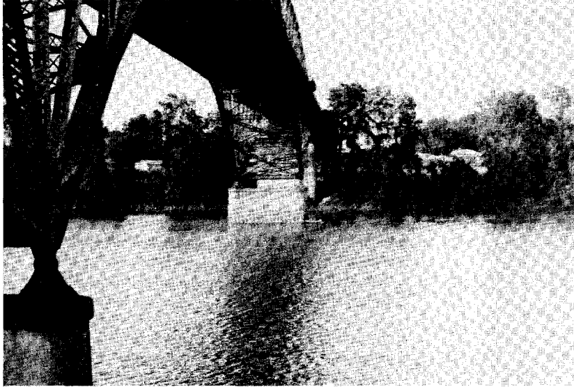
Figure 76. Instrumented Pier #6, Texas Street Bridge over Red River.
