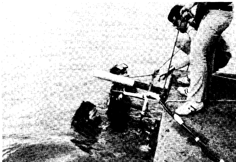
Figure 124. Lowering of package over the side of the footing.
