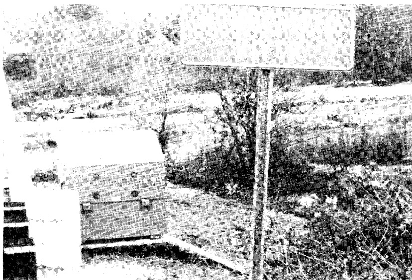
Figure 114. Location of instrumentation housing on downstream side of right abutment.
