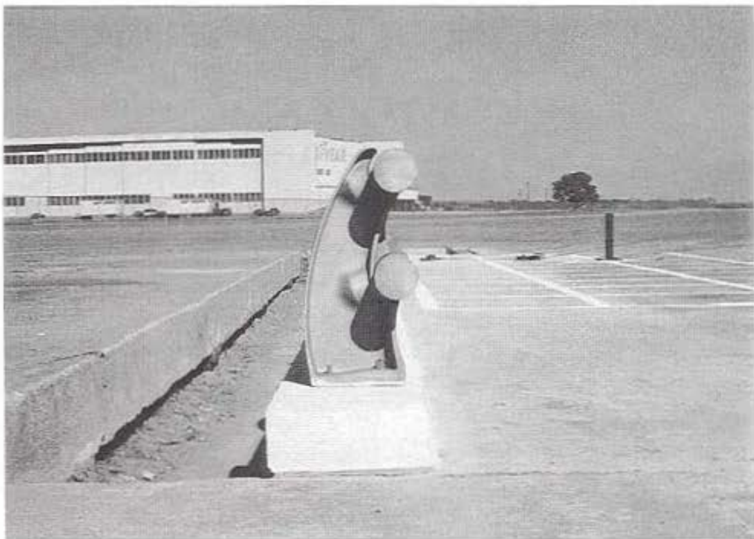
Figure 64. The Foothills Parkway Bridge Rail (continued).
