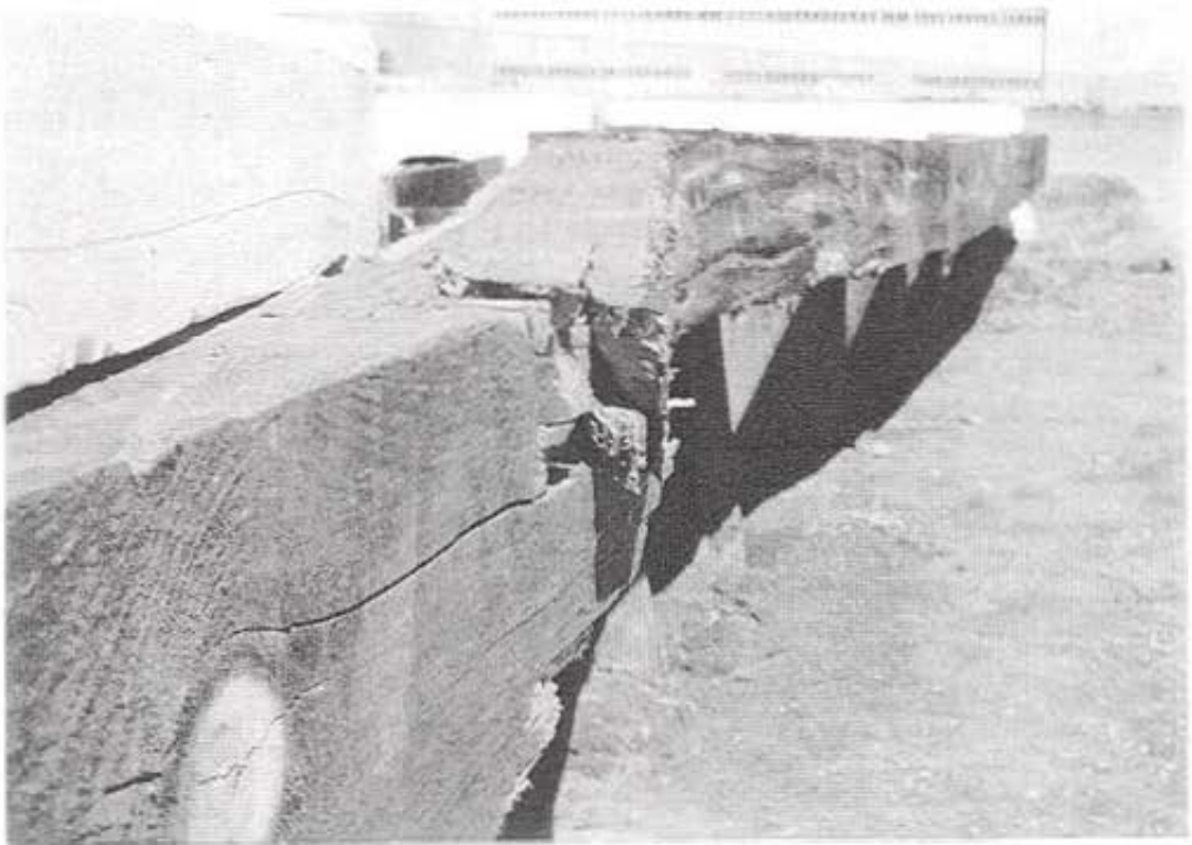
Figure 8. System Damage, Test SBT-1 (continued).
