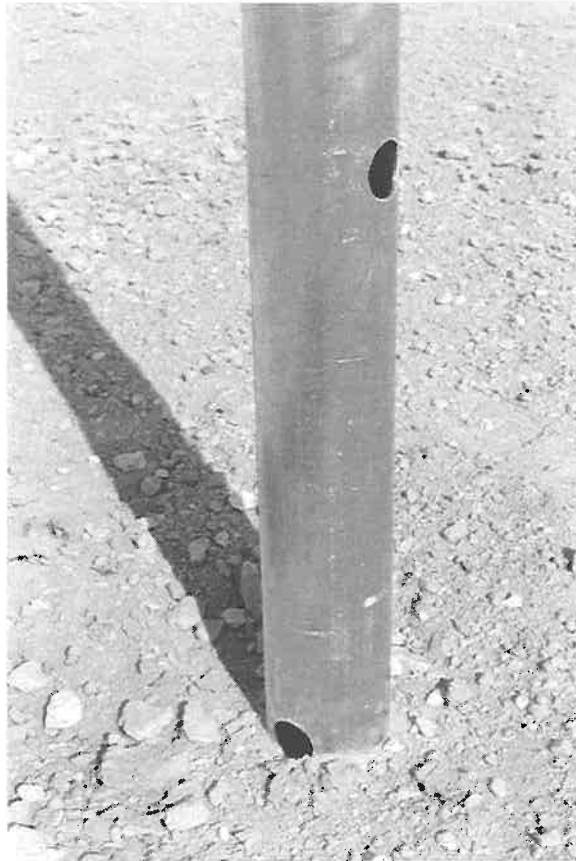
Figure 106. Dual 4 in. aluminum sign support installation modified with four - 1.5 in holes and anchored in strong soil before test 405231-17 (continued).
