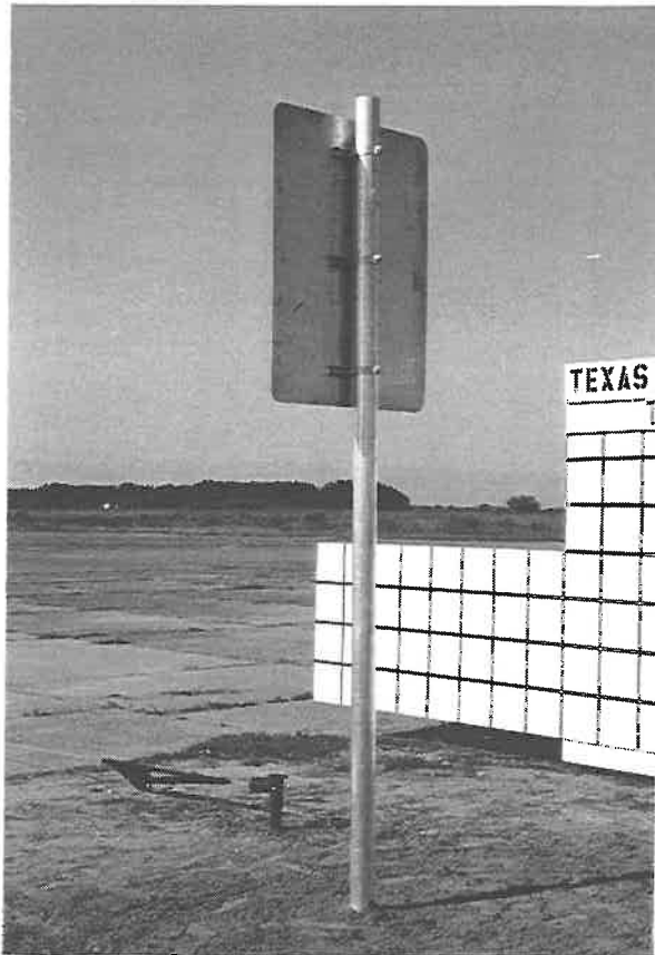
Figure 56 . Single 4 in. aluminum sign support installation anchored in weak soil before test 405231-8.
