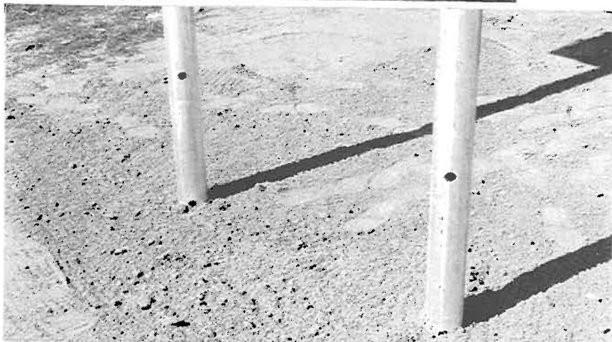
Figure 169 . Dual 4-in with 1-in holes aluminum sign support anchored in weak soil before test 405231-26.
