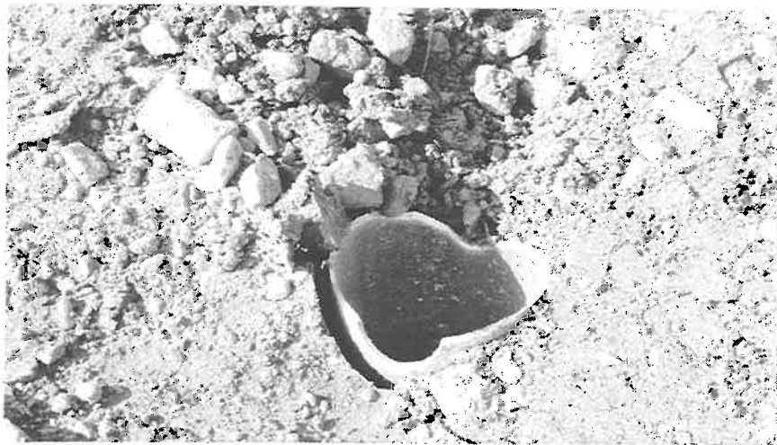
Figure 101. Dual 4 in. aluminum sign support installation modified with four - 1.5 in. holes and anchored in strong soil after test 405231-16.
