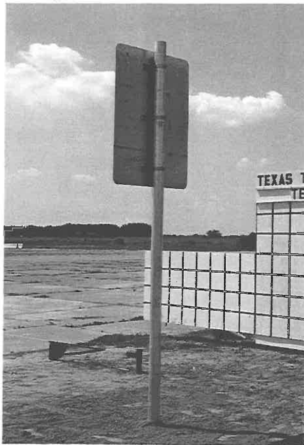
Figure 62 . Single 4 in. aluminum sign support installation anchored in weak soil before test 405231-9.
