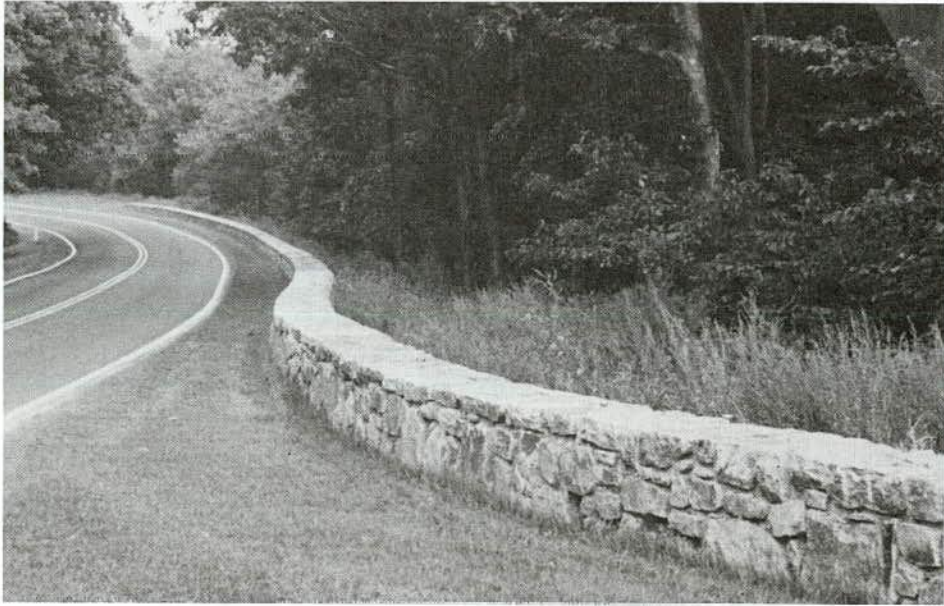
FIGURE 65 Stone masonry guardwall—Skyline Drive, Virginia.
