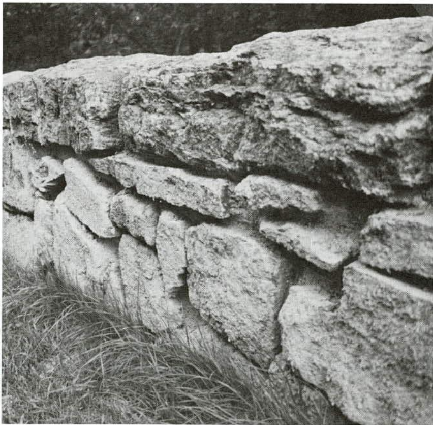
FIGURE 66 Closeup of a stone masonry guardrail.
