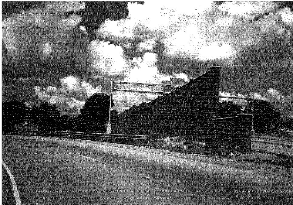
Figure 104: Brick Sound Wall (Jefferson County, I-264)
