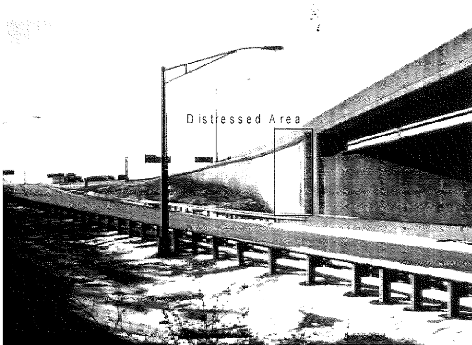
Figure 94a: Distressed Area on M.S.E. Wall (Kenton County, Wall # 2)
