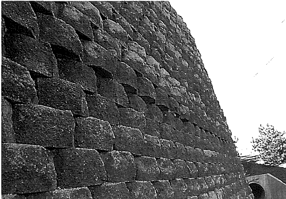
Figure 65a: Forward Displacement between Rows (sliding)
