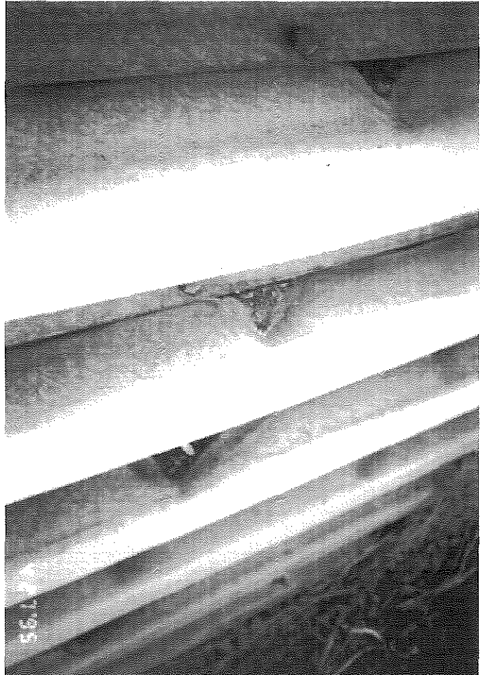
Figure 33: Bending in Horizontal Crib Members
