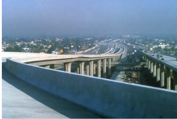
Figure 4-44. I-105 to I-110 Managed Lane Ramp in Los Angeles, California.
