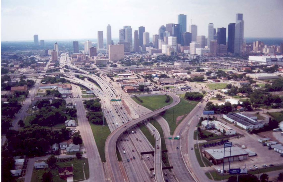
Figure 4-36. Photograph of Flyover Ramp at Downtown Terminus of I-45 (Gulf Freeway) in Houston, Texas.
