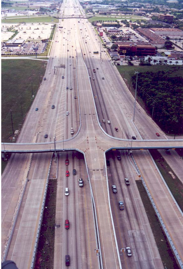
Figure 4-27. Access to Two Park-and-Ride Facilities along I-45 (Gulf Freeway) in Houston, Texas.
