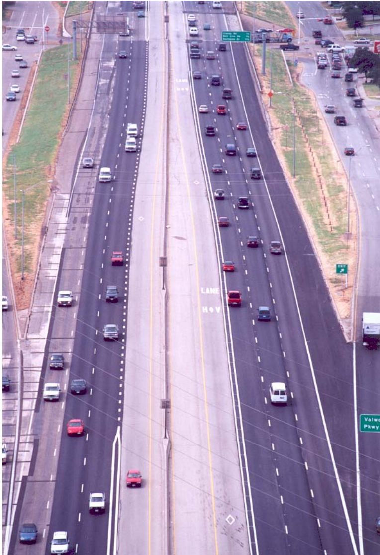
Figure 4-46. I-35E (Stemmons Freeway) Showing Ingress/Egress at the Same Location in Dallas, Texas. (HOV lane access is shown for the downward direction of the HOV lane)
