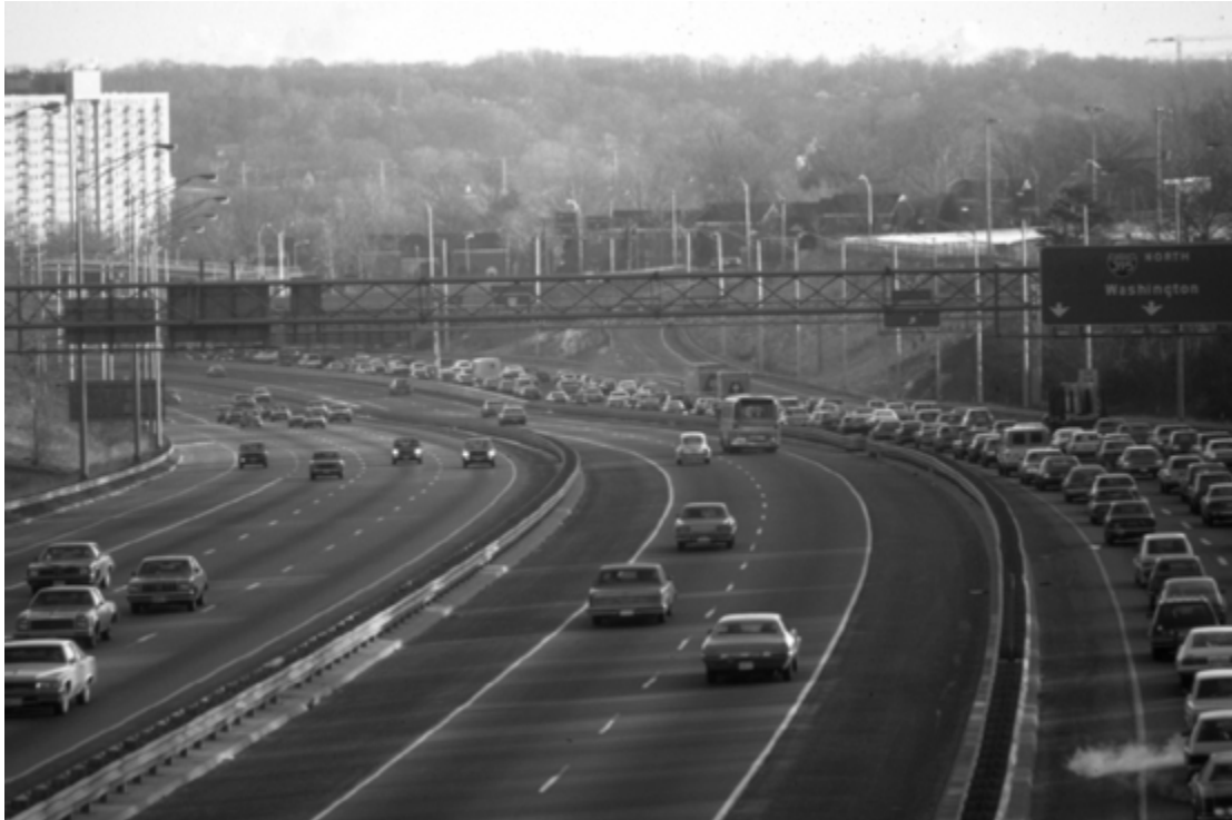
Figure 3-7. Shirley Highway HOV Lanes in Northern Virginia/Washington, D.C.
