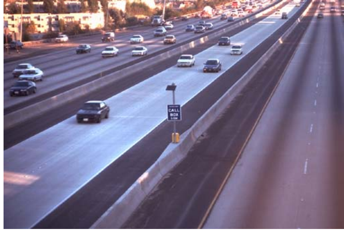
Figure 3-5. Two-Lane Reversible Facility with Call Box on I-15 in San Diego, California.
