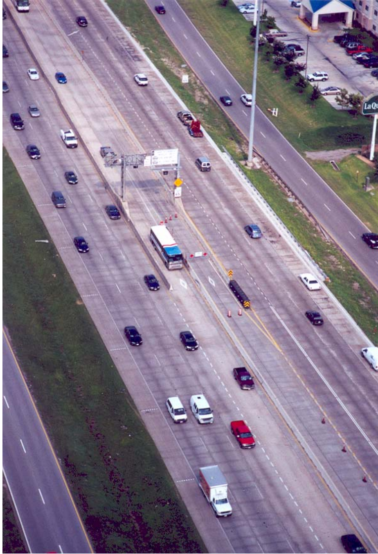
Figure 4-60. Slip Ramp from Barrier-Separated to Concurrent Flow Facility on I-10 (Katy Freeway) in Houston, Texas.
