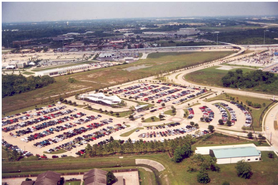
Figure 3-23. Fuqua Transit Station and Park-and-Ride Lot along I-45 (Gulf Freeway) in Houston, Texas.
