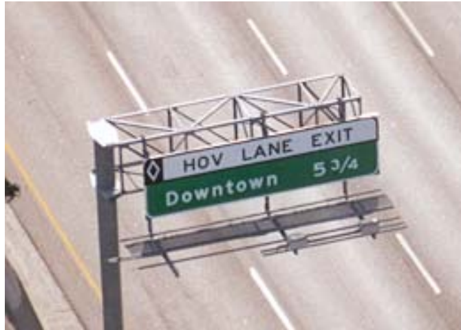
Figure 5-7. Overhead Exit Signing on I-30 (East R. L. Thornton Freeway) in Dallas, Texas.
