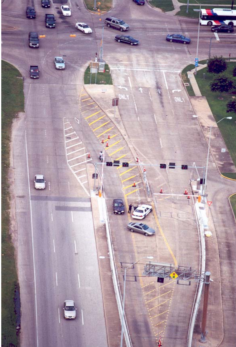
Figure 3-29. Enforcement of 3+ Operation at Entrance to I-10 (Katy Freeway) HOV Lane in Houston, Texas.
