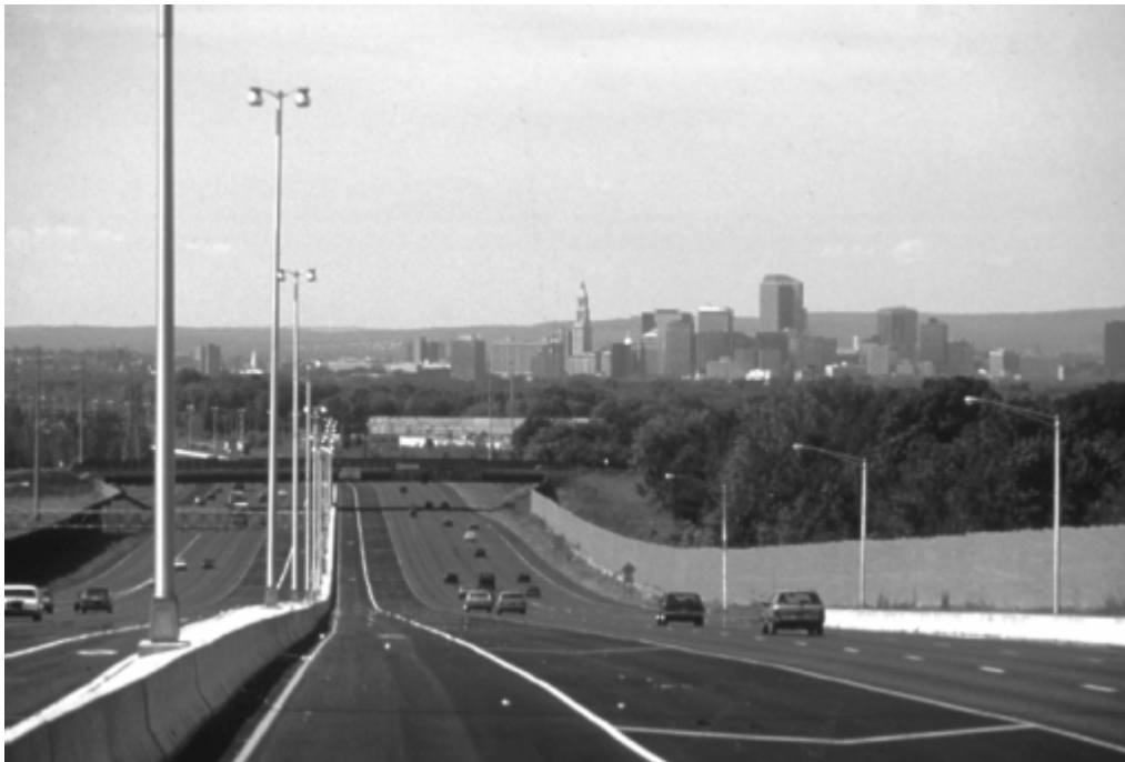
Figure 3-3. I-84 Freeway HOV Lanes in Hartford, Connecticut.
