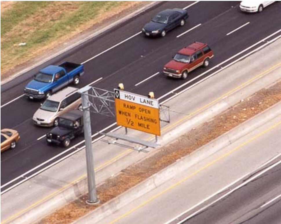
Figure 5-2. Advance Signing on I-35E (Stemmons Freeway) in Dallas, Texas.
