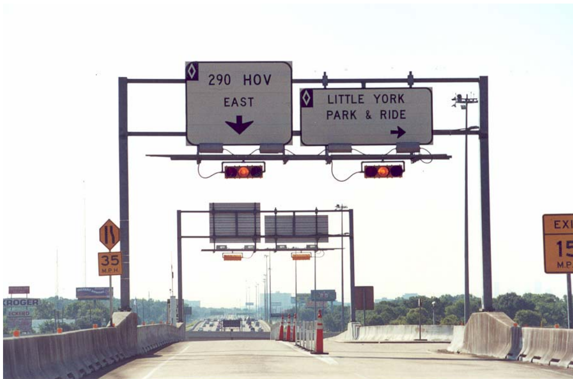
Figure 5-6. Overhead Signing on Reversible HOV Facility at Park-and-Ride Lot on US 290 (Northwest Freeway) in Houston, Texas.
