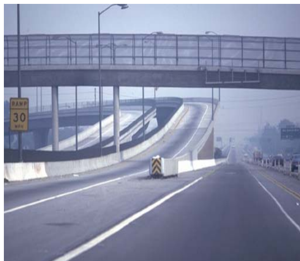
Figure 4-39. Flyover Ramps at Del Mar Avenue on I-10 (El Monte) in Los Angeles, California.
