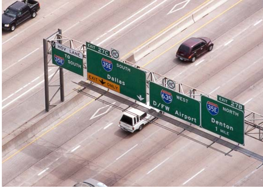
Figure 5-4. Advance Signing for HOV Lane on I-635 (LBJ Freeway) in Dallas, Texas.
