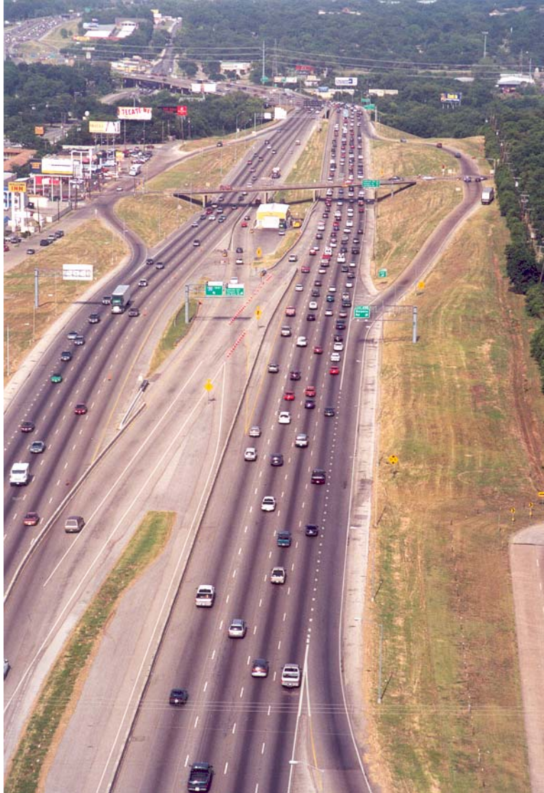
Figure 4-59. X-ramp of Afternoon Operation Showing Exit Ramp to Upward Direction General-Purpose Near Dolphin Road on I-30 (East R. L. Thornton Freeway) in Dallas, Texas. (HOV lane makes an “S” curve through the middle of the X-ramp)
