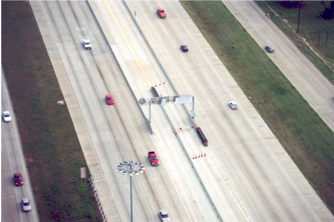
Figure 3-18. Slip Ramp along I-45 (North Freeway) in Houston, Texas.
