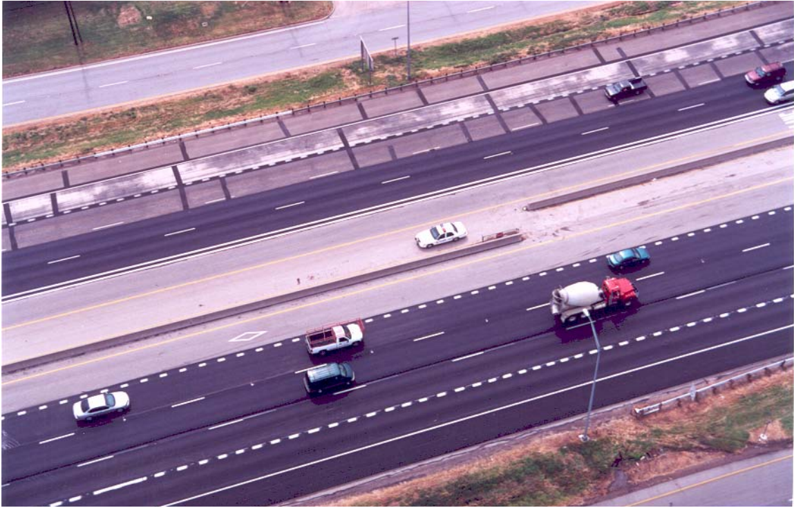
Figure 3-26. Enforcement Zone with Police Vehicle Showing Gate for Bi-Directional Enforcement on I-35E (North Stemmons) in Dallas, Texas.
