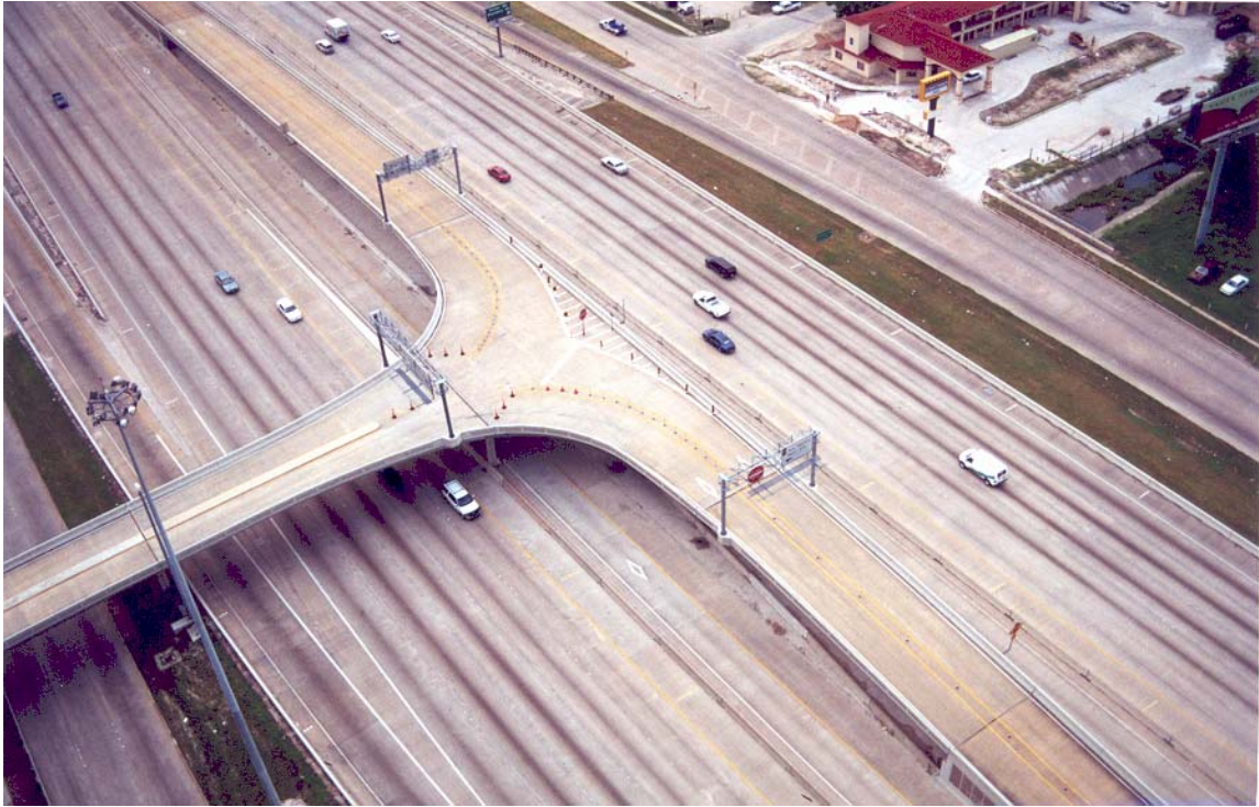
Figure 4-25. Design Features of T-ramp with Entrance/Exit Features along US 59 (Eastex Freeway) in Houston, Texas. (Through traffic handled at ground level)
