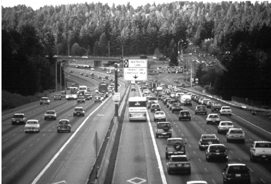
Figure 3-9. I-5 North Concurrent Flow HOV Lanes in Seattle, Washington.
