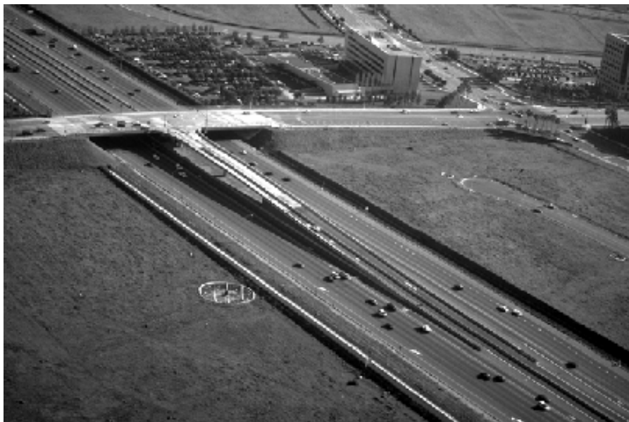
Figure 3-15. Drop Ramp in Orange County, California. (Managed flow main lane continues under overcrossing road)
