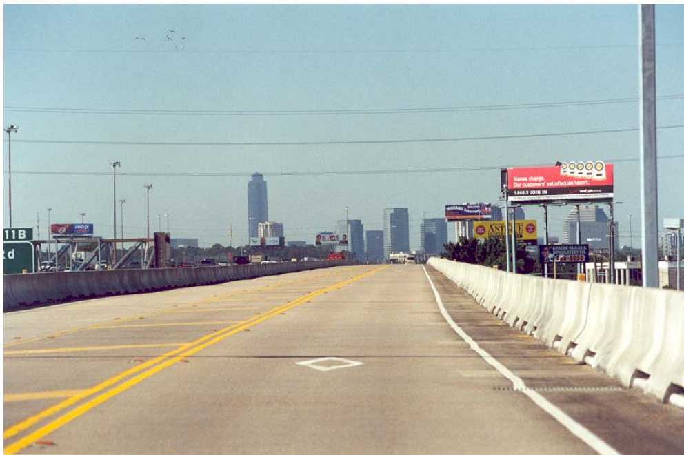
Figure 5-12. Diamond Pavement Marking on US 290 (Northwest Freeway) Terminus to Northwest Transit Center.
