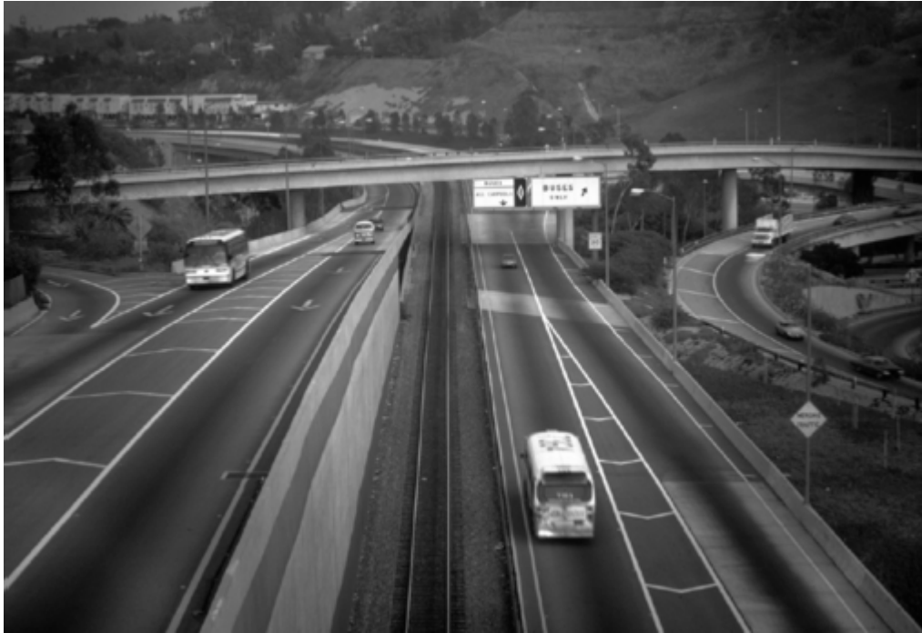
Figure 3-2. San Bernardino Transitway in Los Angeles, California.
