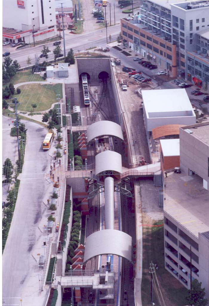
Figure 2-2. Intermodal Station at Mockingbird in Dallas, Texas. (local bus parking [left] and rail tunnel)
