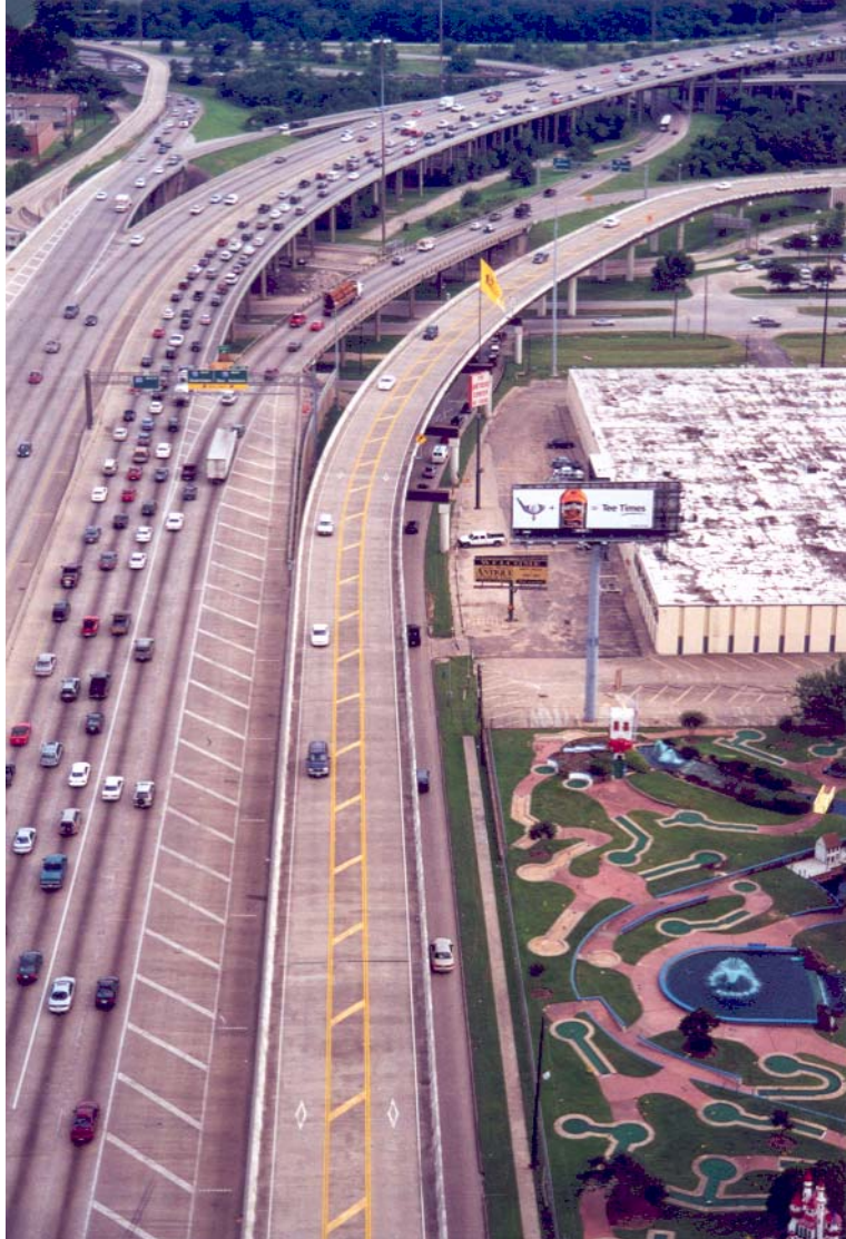
Figure 4-41. Two-way Elevated Flyover along I-610/ US 290 in Houston, Texas.
