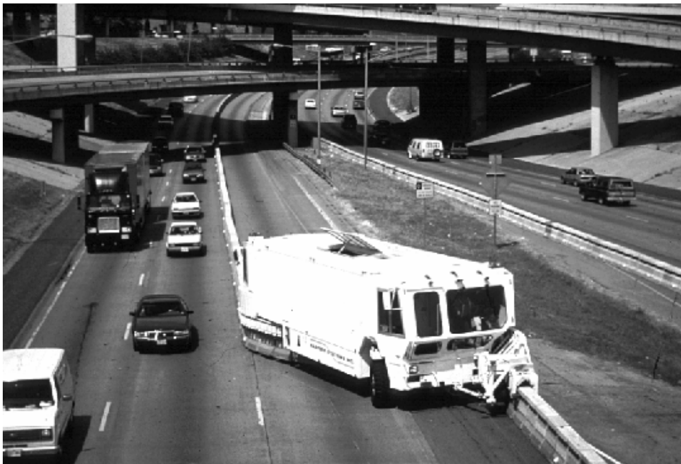
Figure 3-12. Moveable Barrier and Contraflow HOV Lane on I-30 (East R. L. Thornton Freeway) in Dallas, Texas.
