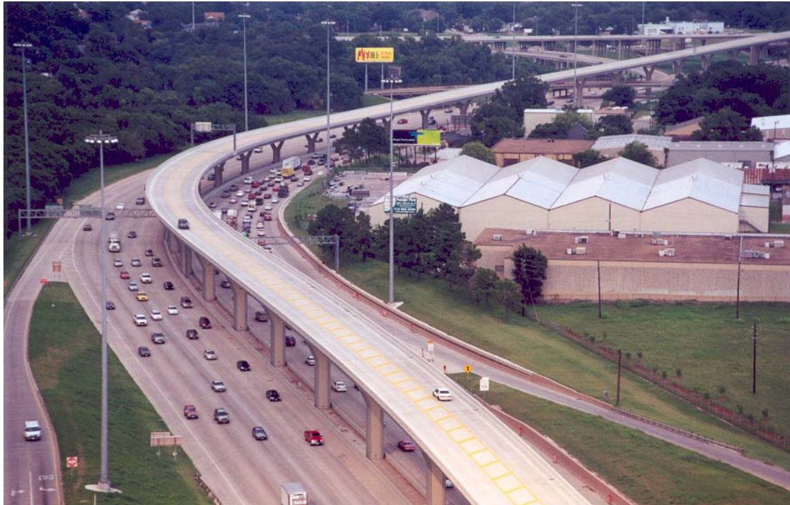
Figure 4-42. Two-way Elevated Flyover along I-10 (Katy Freeway) in Houston, Texas.
