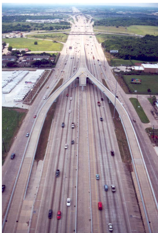
Figure 4-34. Wishbone Flyover Ramp at Dixie Farm Road at Southern End of I-45 (Gulf Freeway) Managed Lane in Houston, Texas.
