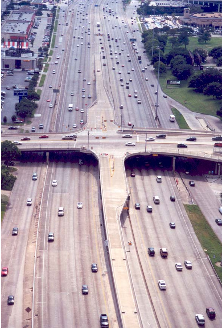
Figure 4-30. Drop Ramp at Edloe on US 59 (Southwest Freeway) in Houston, Texas.
