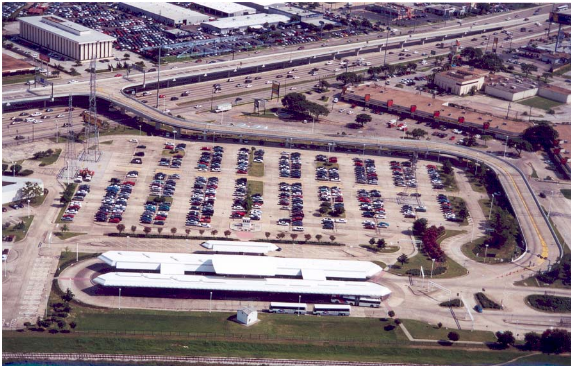
Figure 3-21. Westpark Park-and-Ride Lot along US 59 (Southwest Freeway) in Houston, Texas.
