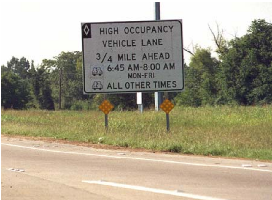
Figure 5-9. Ground-mounted Sign on US 290 (Northwest Freeway) in Houston, Texas.
