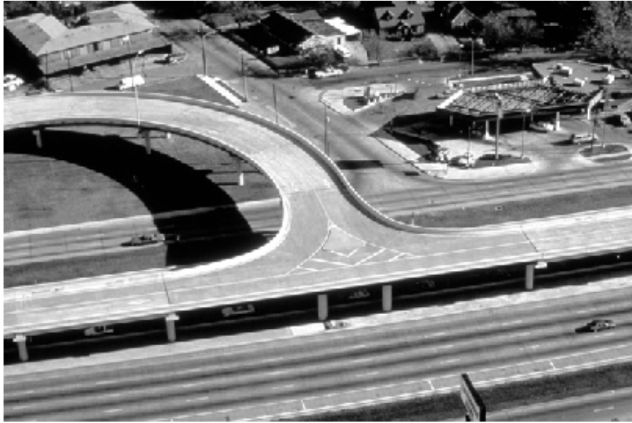
Figure 3-14. T-ramp in Houston, Texas. (Main lane—right to left across photograph, local access ramp toward top)
