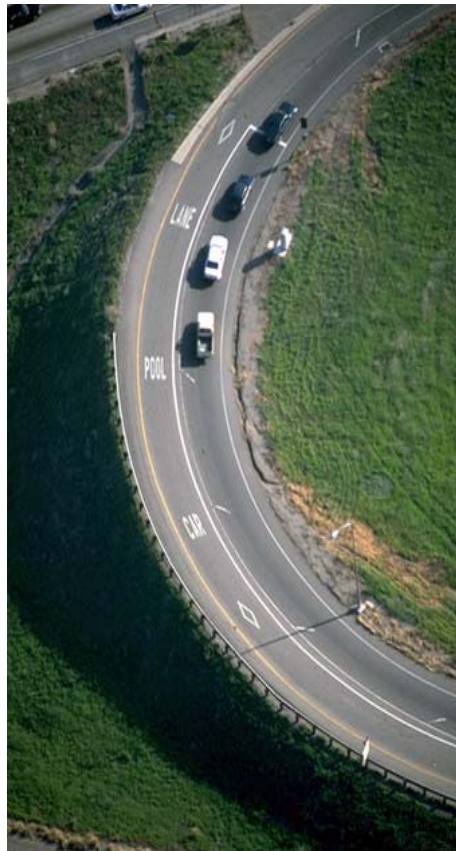
Figure 4-62. Bypass Lane in Los Angeles, California.
