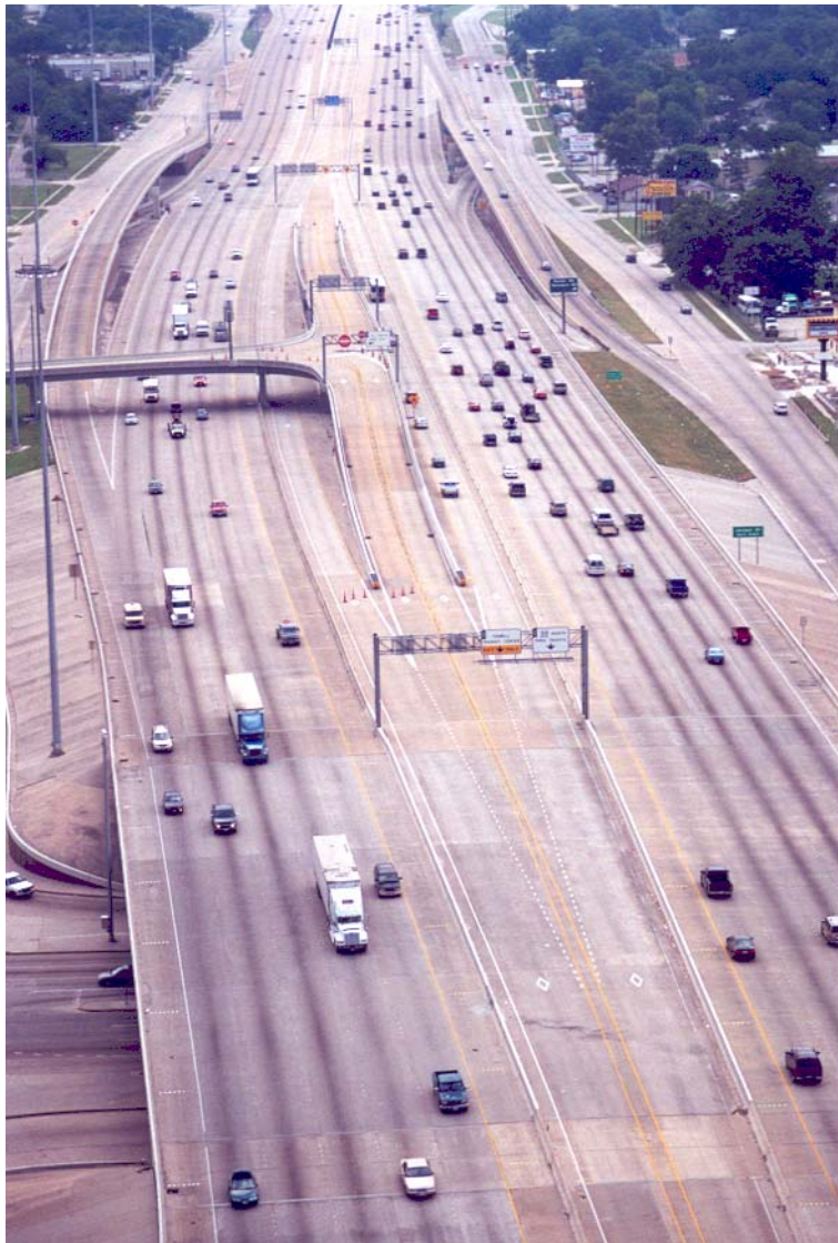
Figure 4-24. T-ramp Transit Center Access with At-Grade Bypass Lanes along US 59 (Eastex Freeway) in Houston, Texas. (Through traffic handled at ground level)
