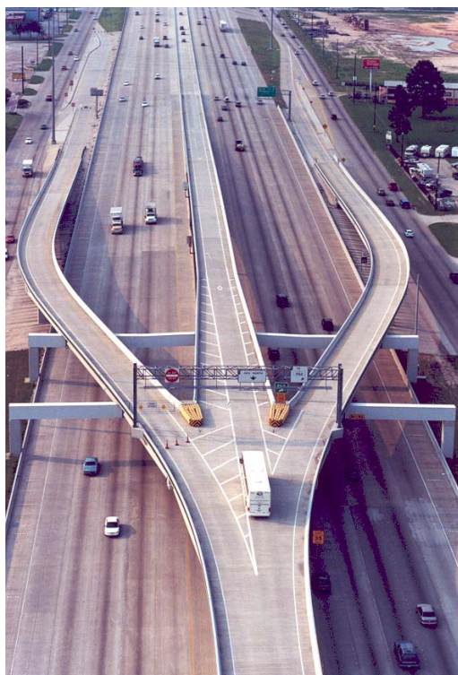
Figure 4-33. Photograph of Flyover Ramp at FM 1960 along I-45 (North Freeway) in Houston, Texas.
