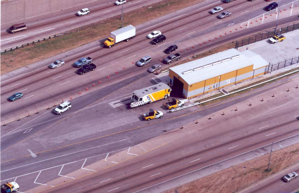
Figure 3-13. Contraflow Lane at Downtown Entrance to I-30E (East R. L. Thornton Freeway) and “Zipper Truck” Used to Move Barriers.
