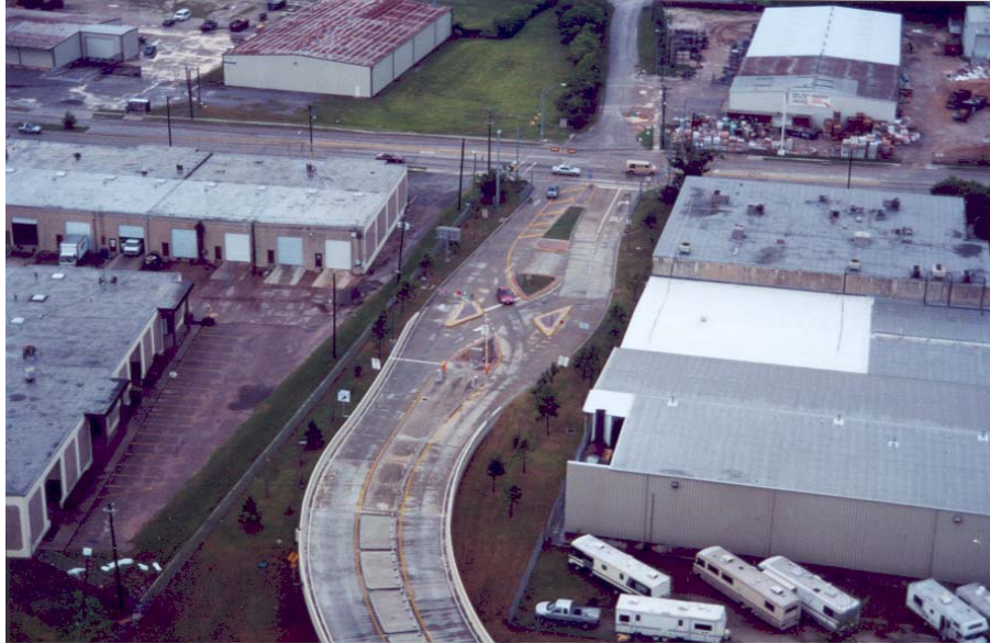
Figure 4-21. Crossover Traffic Operation for T-ramp at an Arterial Street along I-45 (North Freeway) in Houston, Texas.
