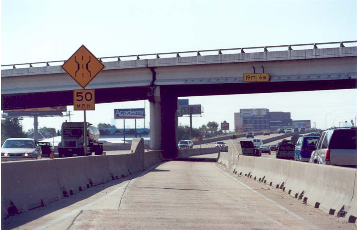
Figure 4-3. Reduced Width along US 290 (Northwest Freeway) Barrier-Separated Facility in Houston, Texas.
