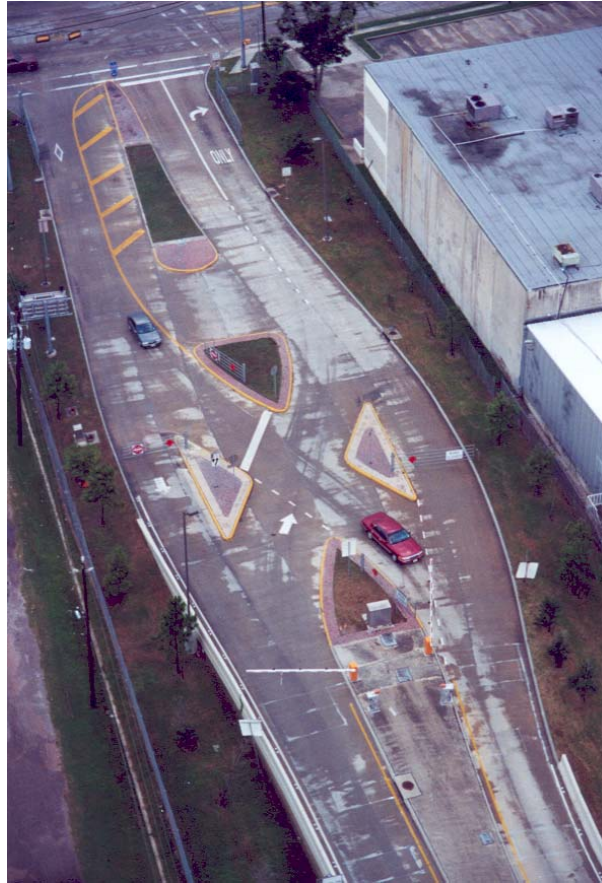
Figure 4-23. Close-up of Ramp Crossover at an Arterial Street along I-45 (North Freeway) in Houston, Texas.
