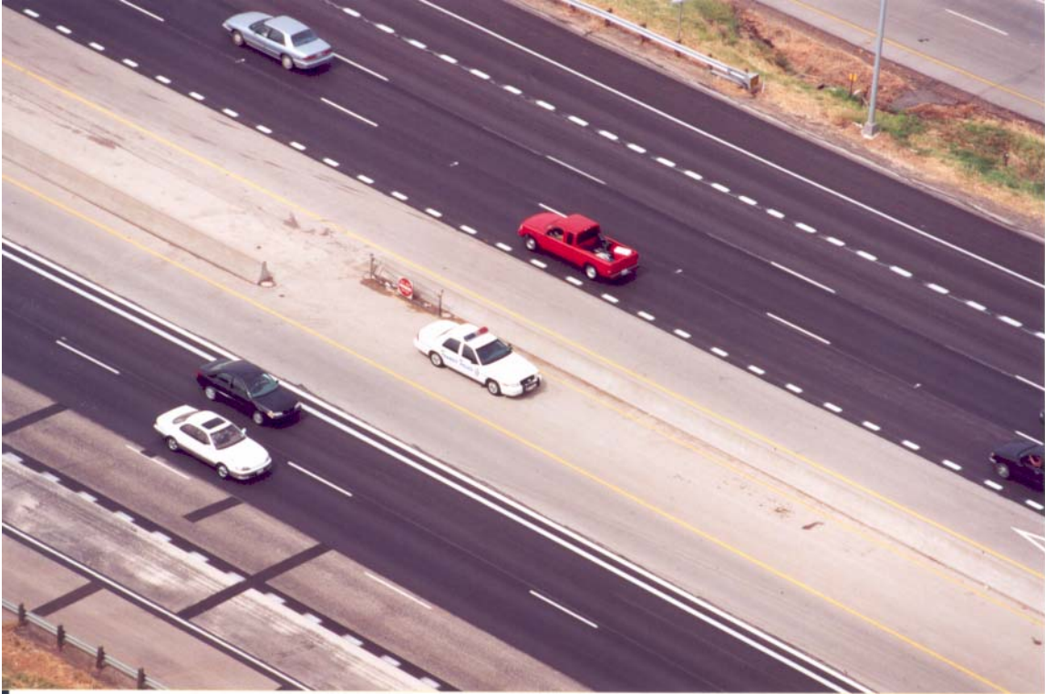
Figure 5-15. Pavement Markings on I-35 (Stemmons Freeway) in Dallas, Texas. (Limited access point indicated by dashed white line)
