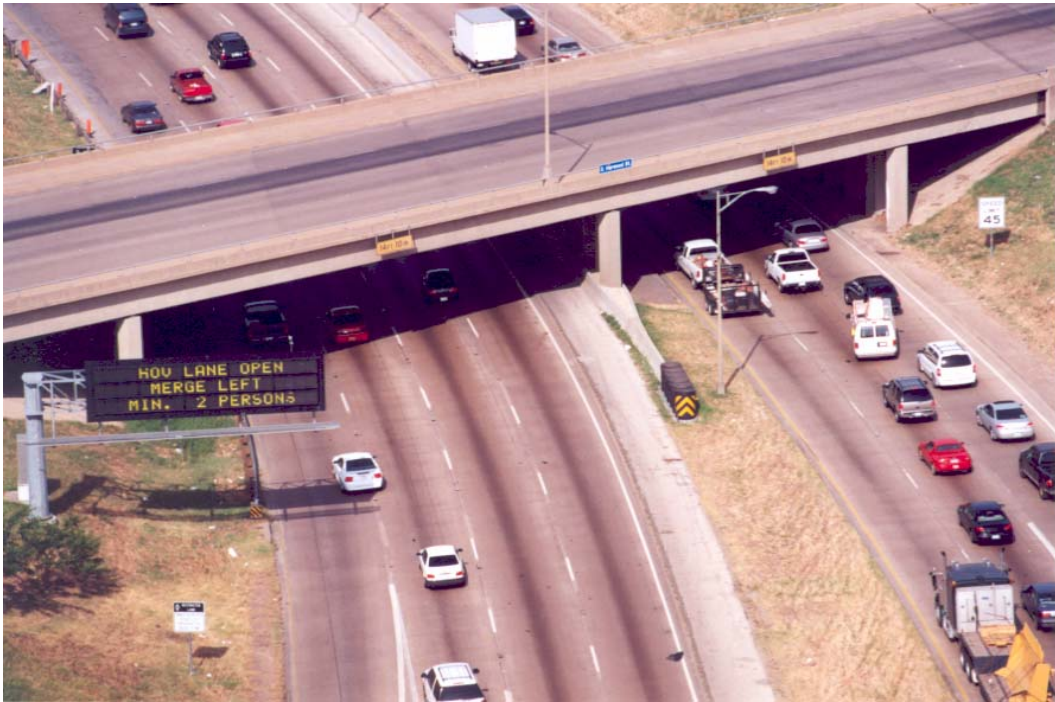
Figure 5-11. Changeable Message Sign on I-30 (East R. L. Thornton Freeway) in Dallas, Texas.
