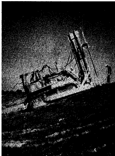
Figure 46. Modified crawler tractors used to inject lime slurry.
