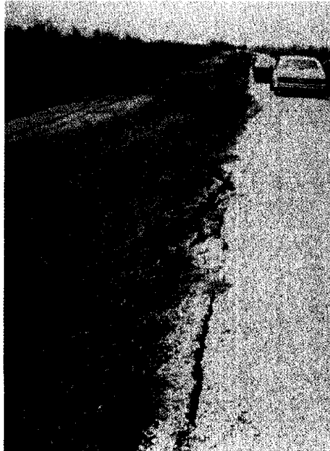
Figure 45. Damaged slope due to failure slides.
