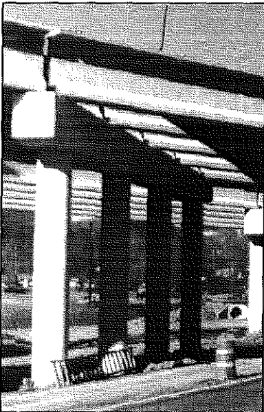
Figure 1.4.2a. Skew Angle of the Girders.
