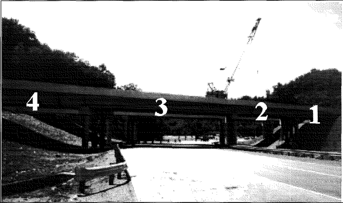
Figure 2.2. US 23 Bridge Over KY 40 (Span Numbers Are Marked - Northbound Traffic Travels from Right to Left [←]).
