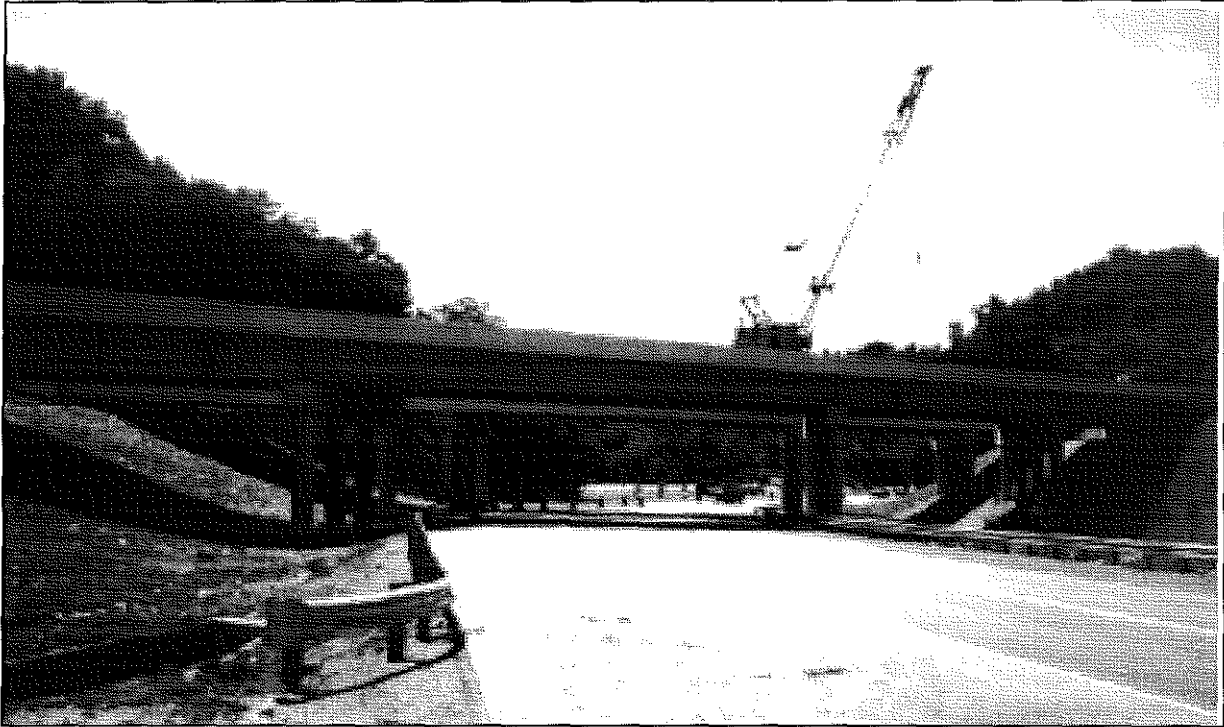
Figure E-1. Southbound and Northbound (foreground) US 23 Bridges Over KY 40
