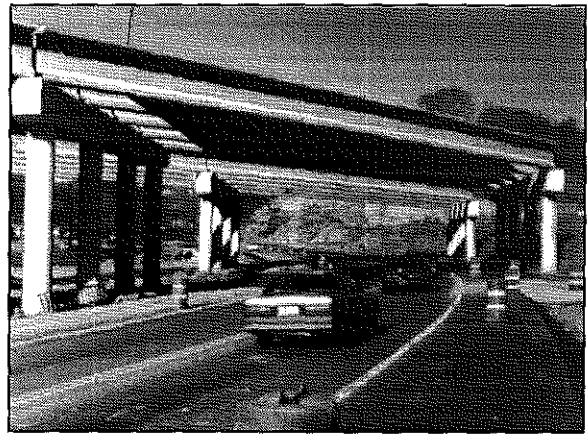
Figure 2.1. Span 3 of the US 23 Bridges.
