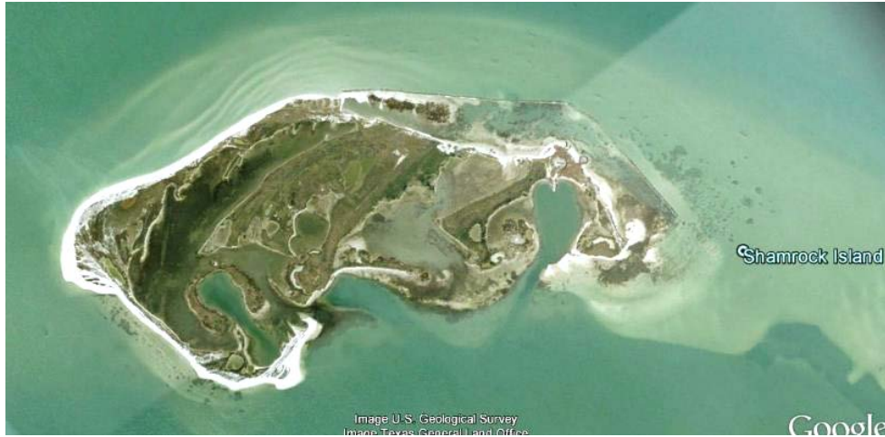
Figure 8. Shamrock Island in 2004 after Installation of Geotextile Tubes on Northeastern Portion.
