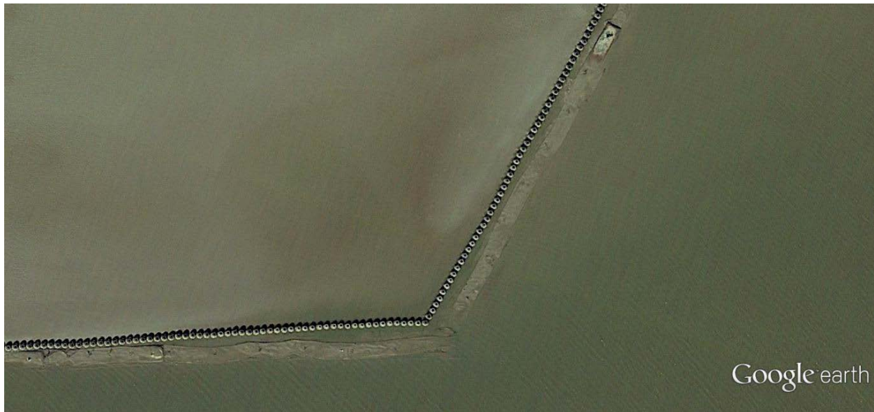
Figure 15. Close-Up of the Geotextile Tubes after 15 Years of Performance in January 2017.
