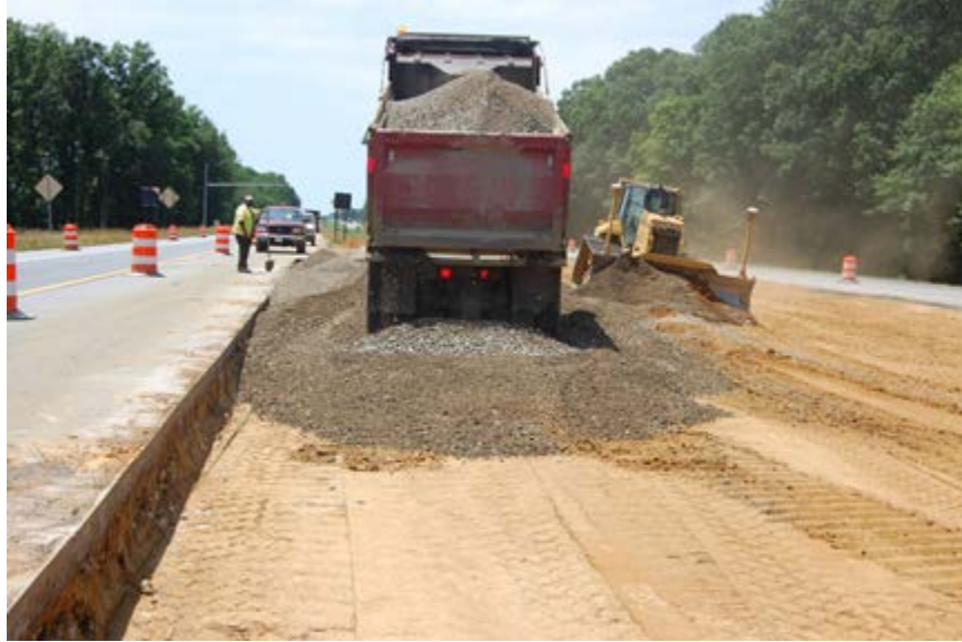
Figure 17. Placement of aggregate stone along Section 2.
