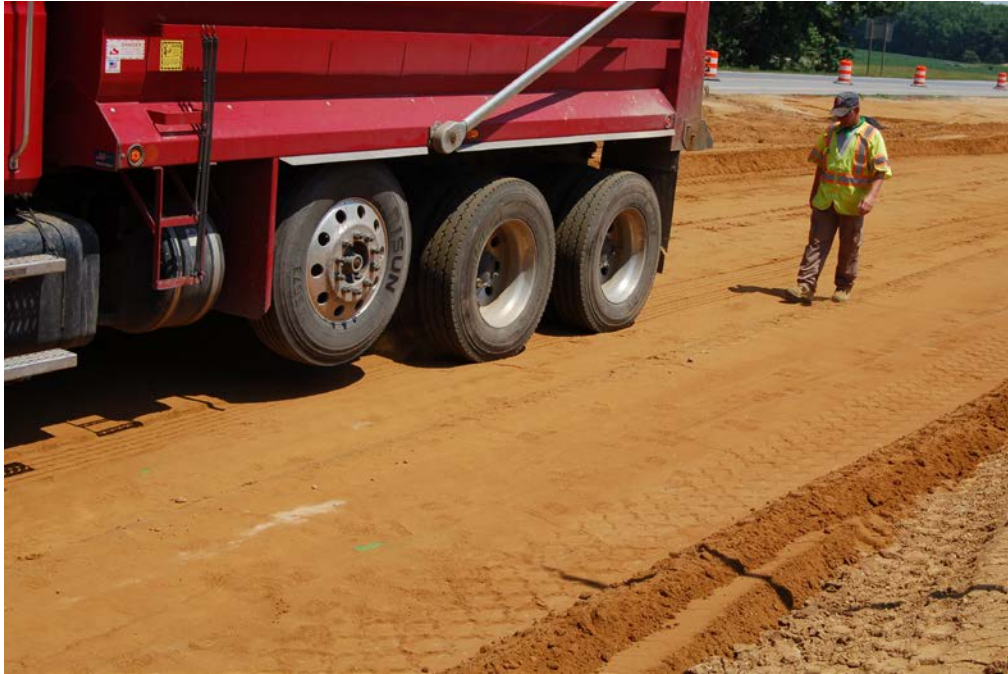
Figure 8. Inspector conducting a proof roll along Section 2.
