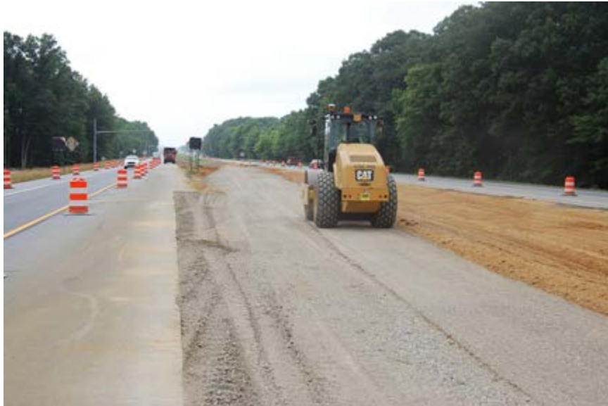
Figure 18. Compaction of aggregate stone along Section 2.
