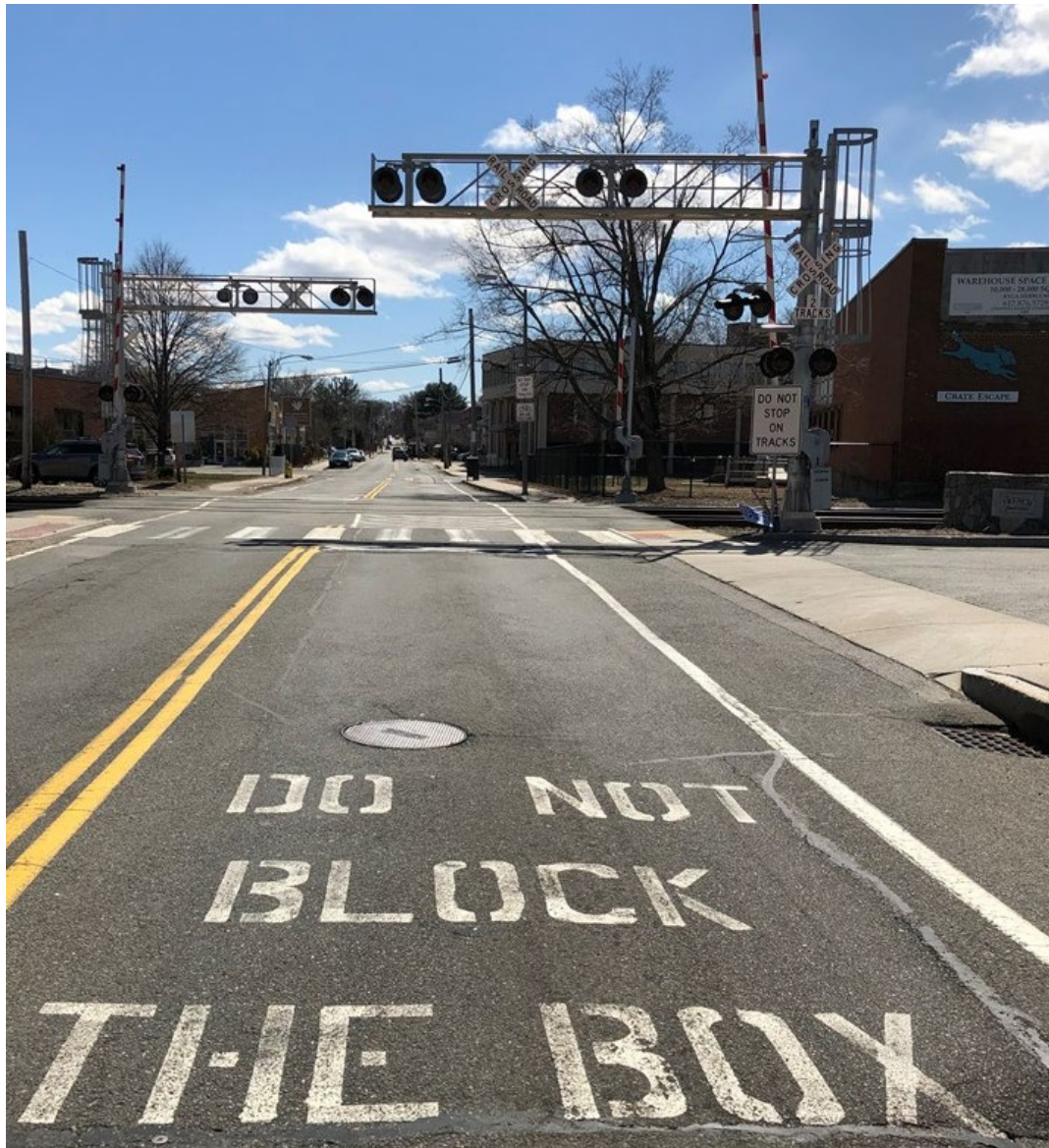
Figure 3. Southbound Approach to the Brighton St. Grade Crossing
