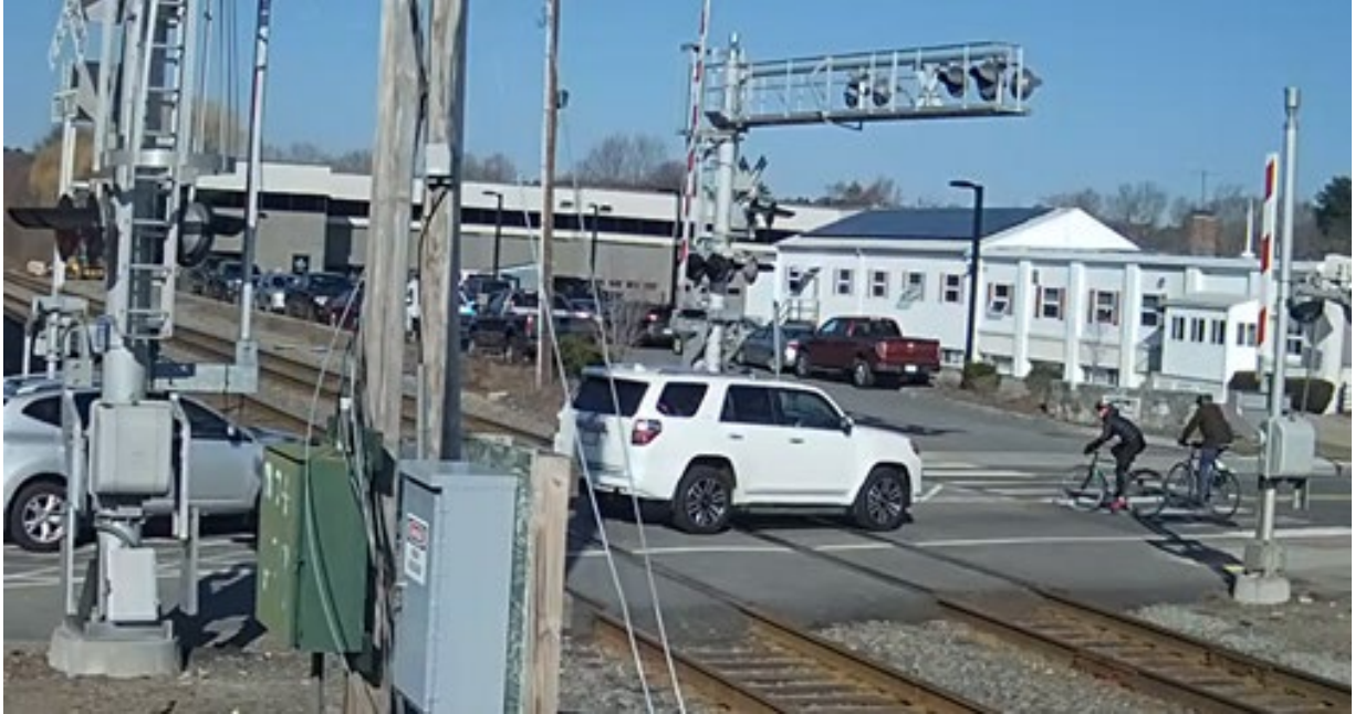
Figure 13. Example of Northbound Vehicles Stopping on Tracks Due to Bicyclists
