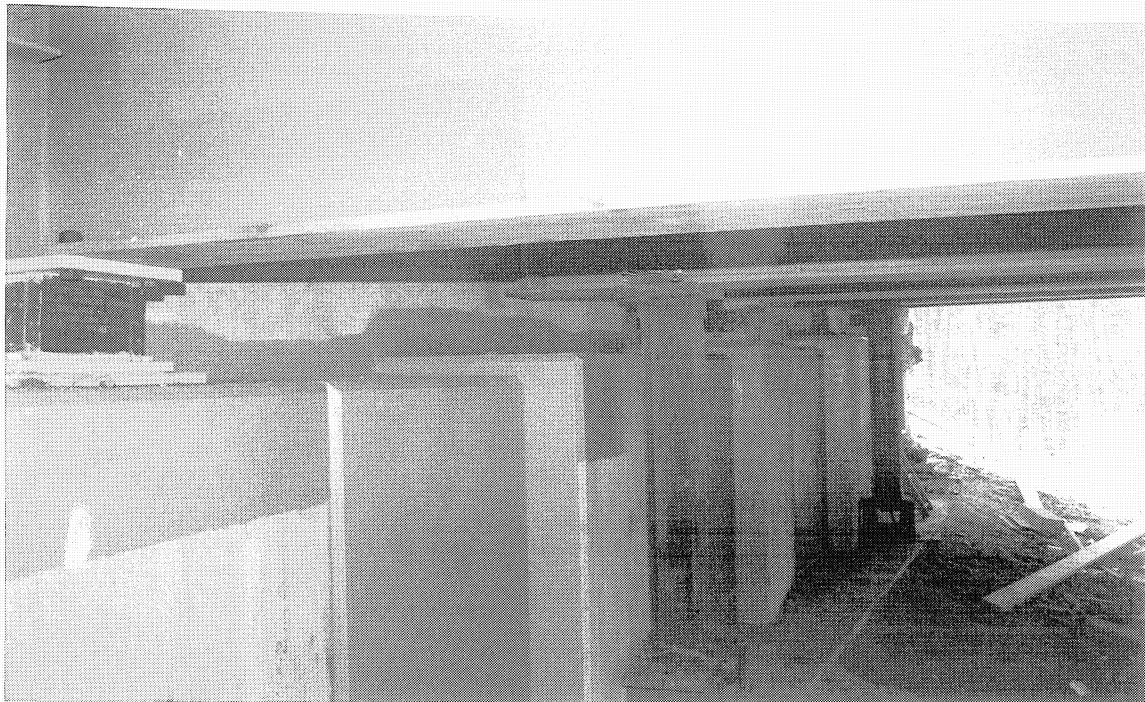
(b) Bearing Installation Procedure at the Abutment
