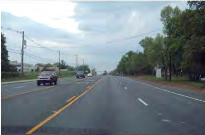
Existing Condition along Route 31
