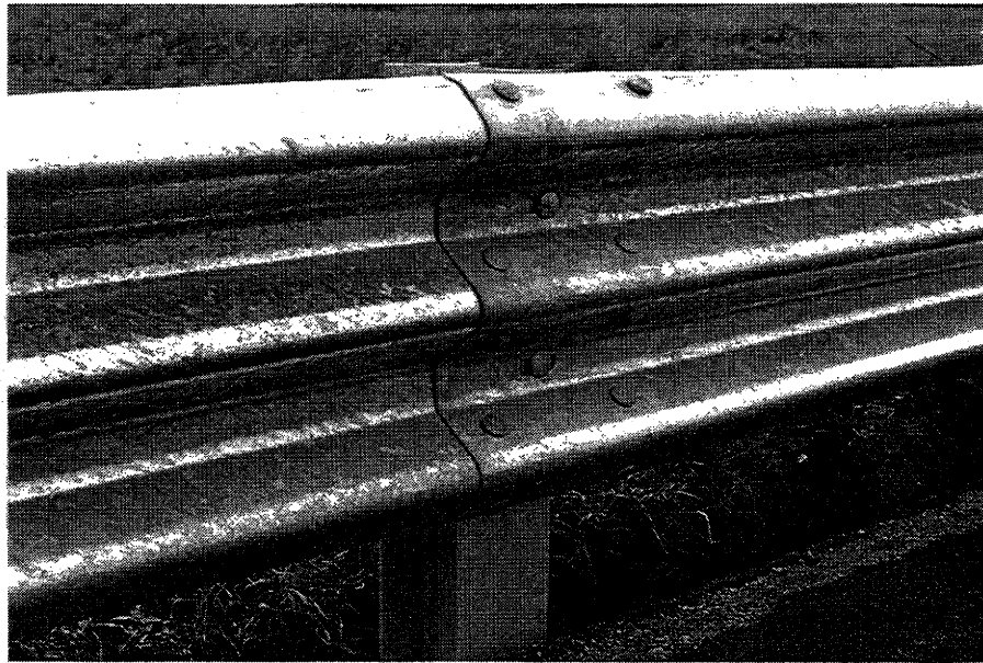
Figure 3. Oregon side-mounted bridge railing (front view) before test 7069-17.
